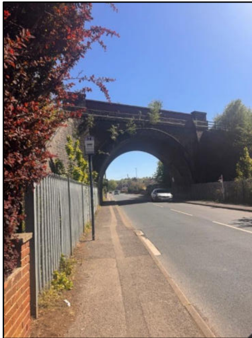
Image 5.3 Existing Bus Stop (Ref: 37055888) located along Cobcar Lane
