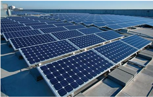
Figure 10. Solar panels installed to flat roof 1
