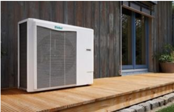
Figure 14. ASHP outdoor unit 5
