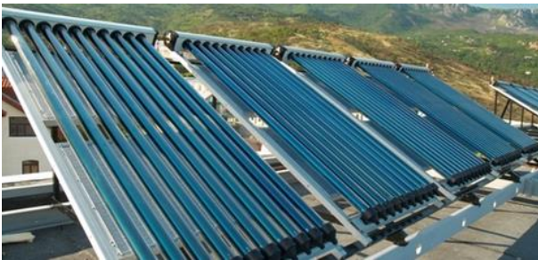
Figure 11. Evacuated tube solar collectors 2
