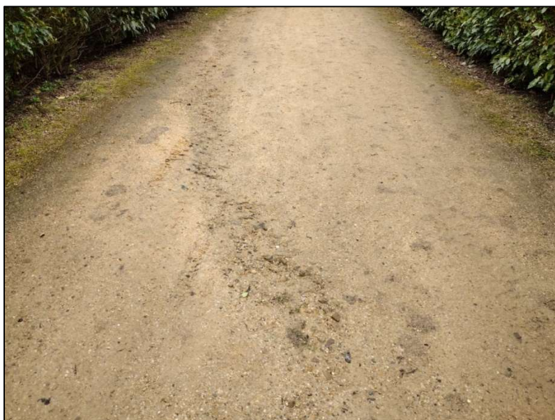
Figure 2: Example of the existing path surface and storm erosion
