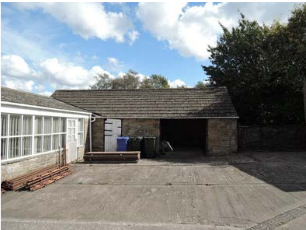
Garage/shed in good order
