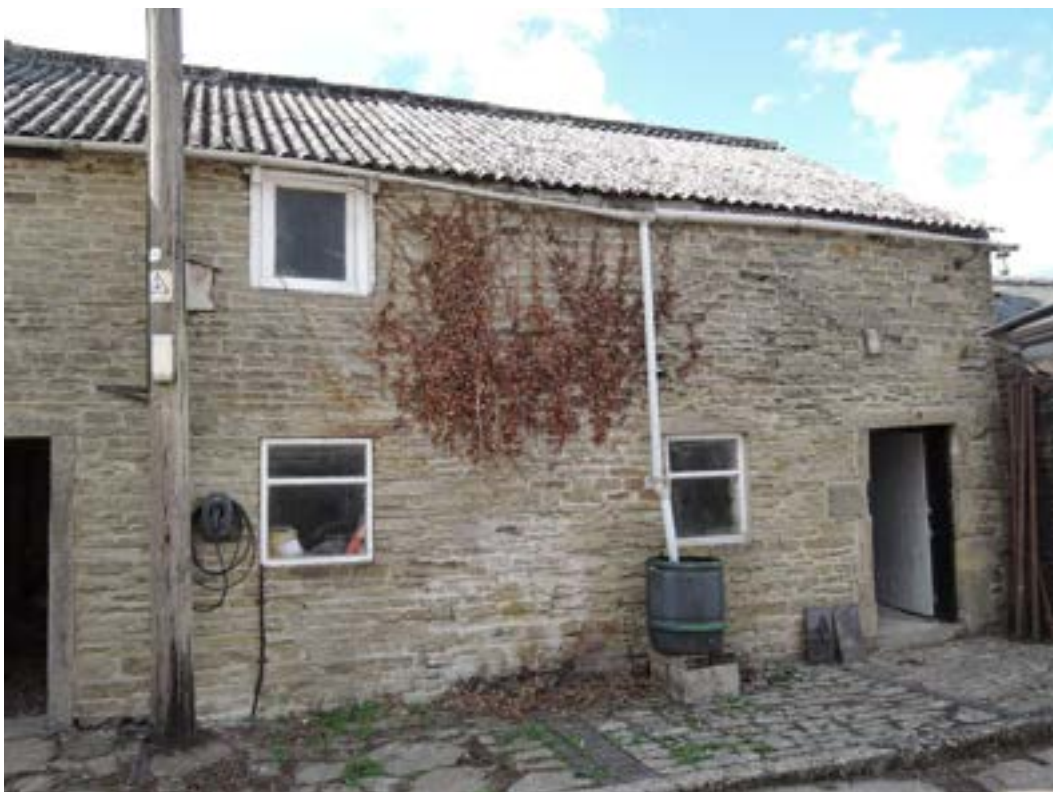
Small barn, yard elevation
