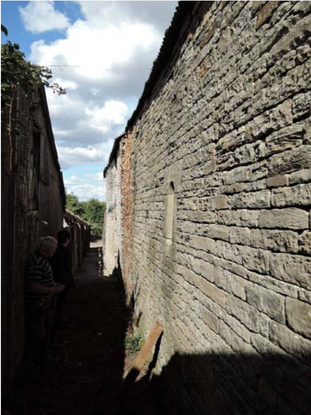
Large barn and small barn back wall back wall looking north
