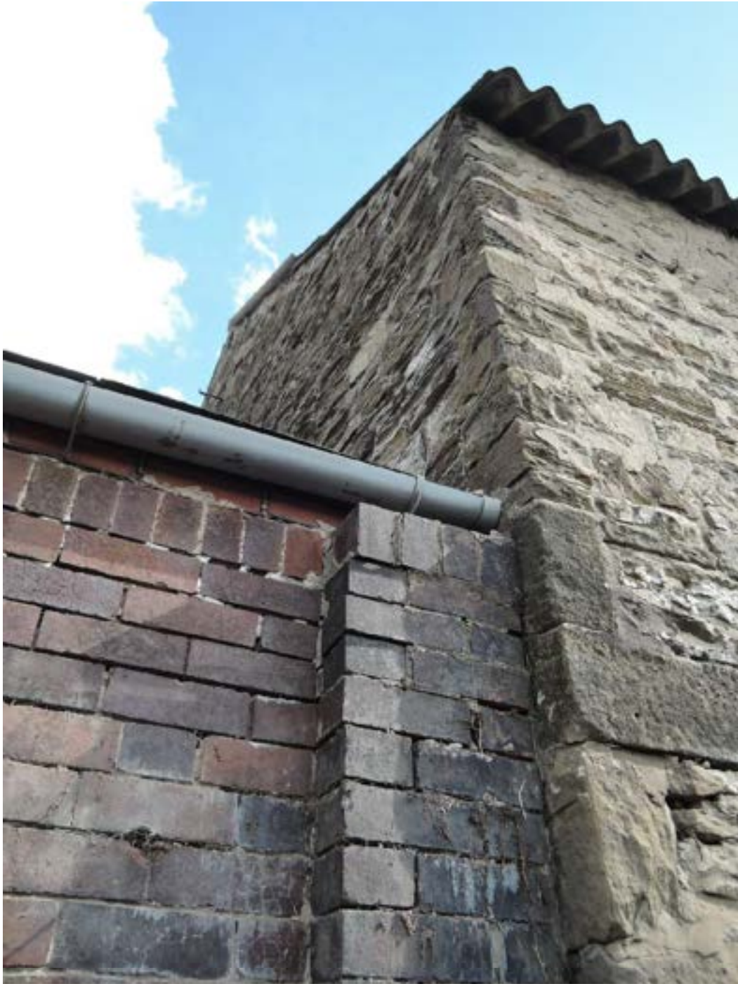
Smaller barn north gable. Brick barn on left to be demolished
