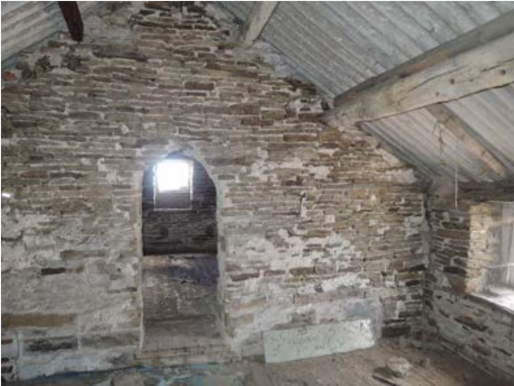
1st floor small barn intermediate wall
