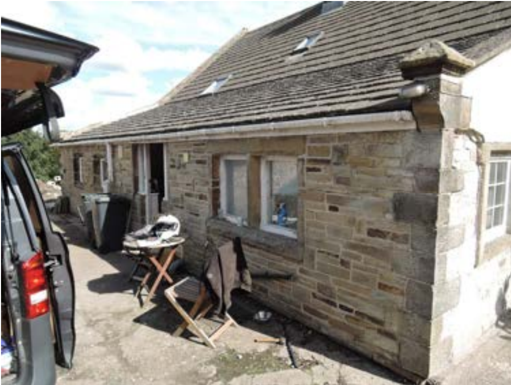
Farmyard side, single storey extension, no signs of distress.
