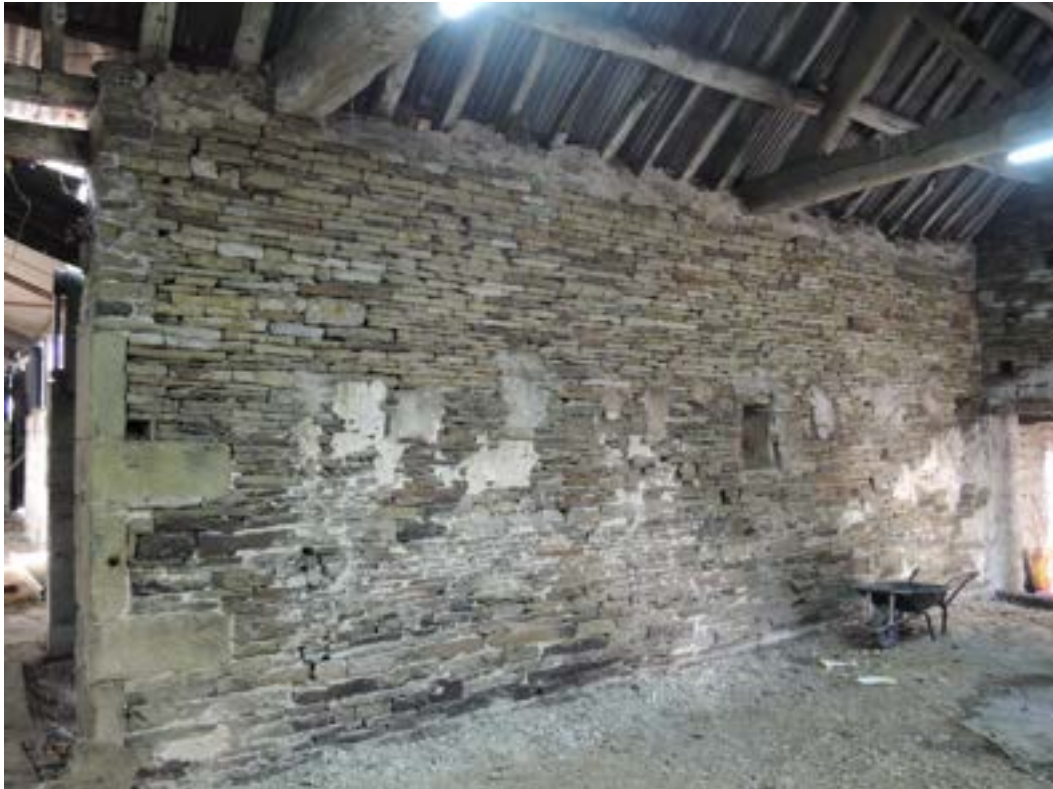
Back wall large barn looking west.
