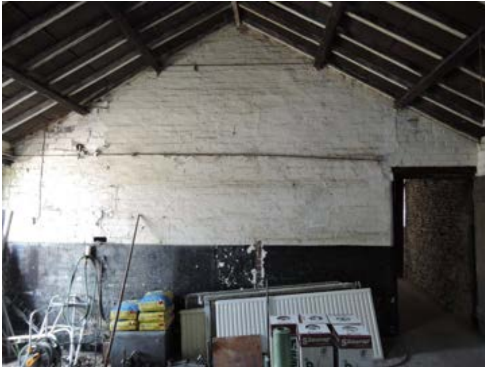
Gable end small barn
