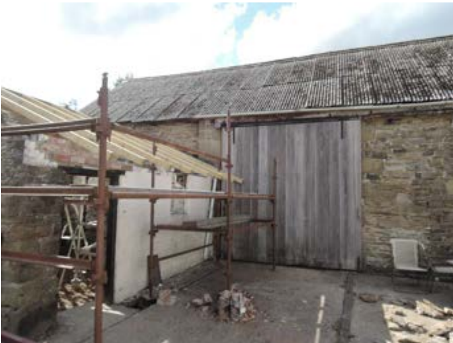
Large barn at south end of yard
