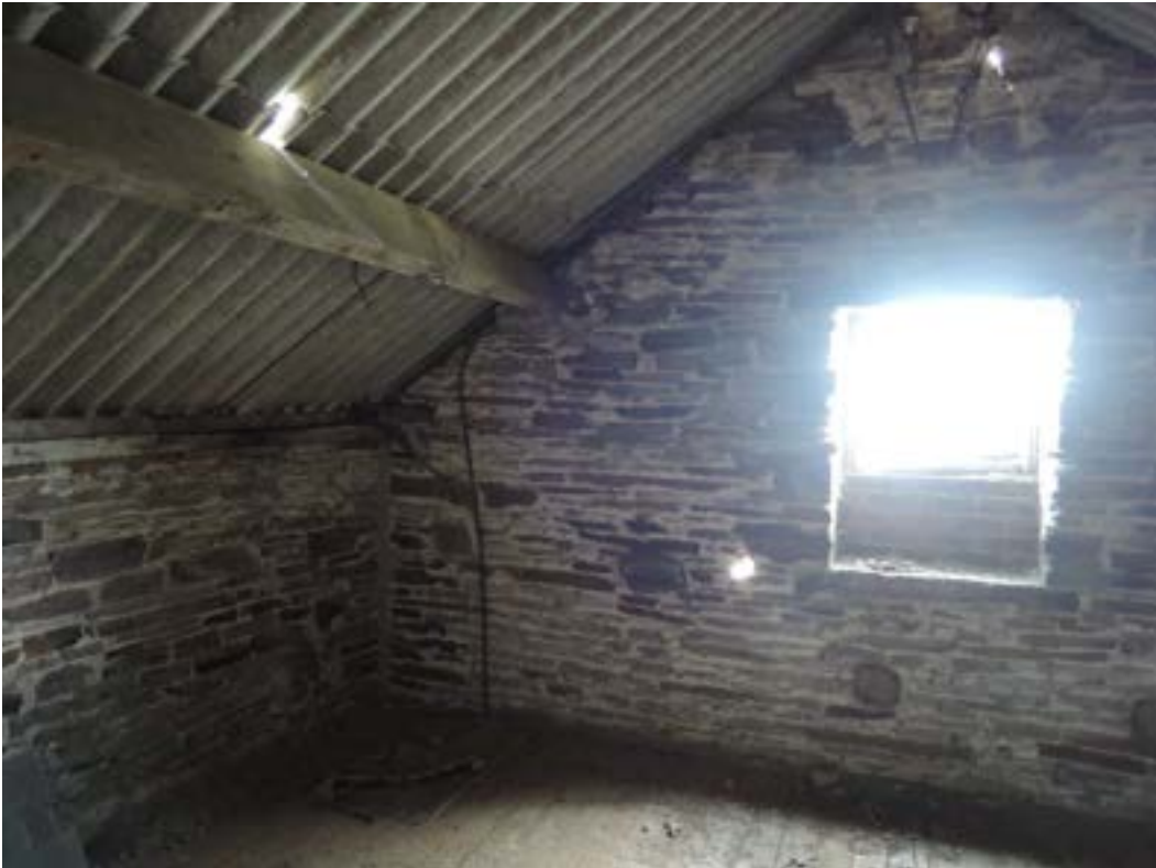
Gable end 1st floor
