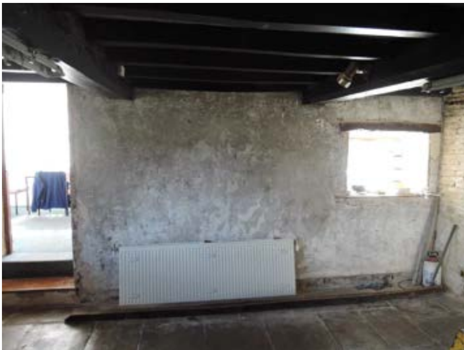
Dining room rear wall looking southwest.
