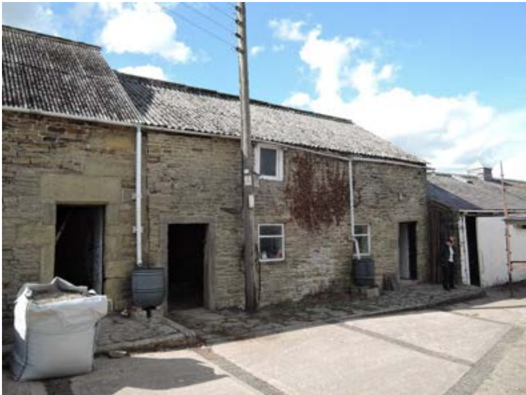
Smaller barn to the north
