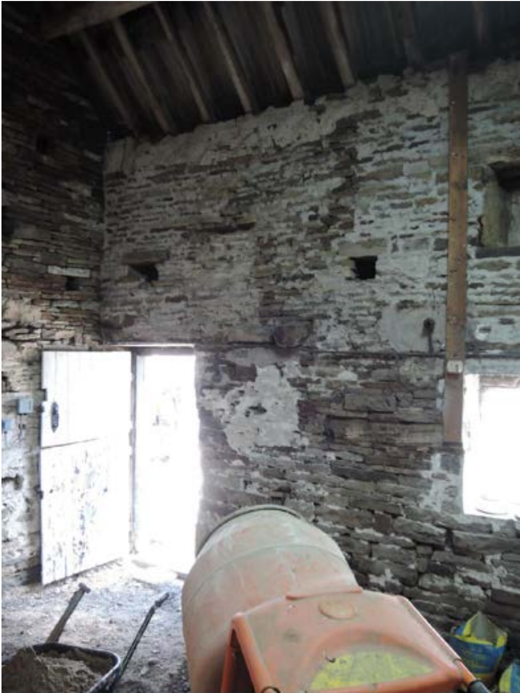
Northeast corner large barn
