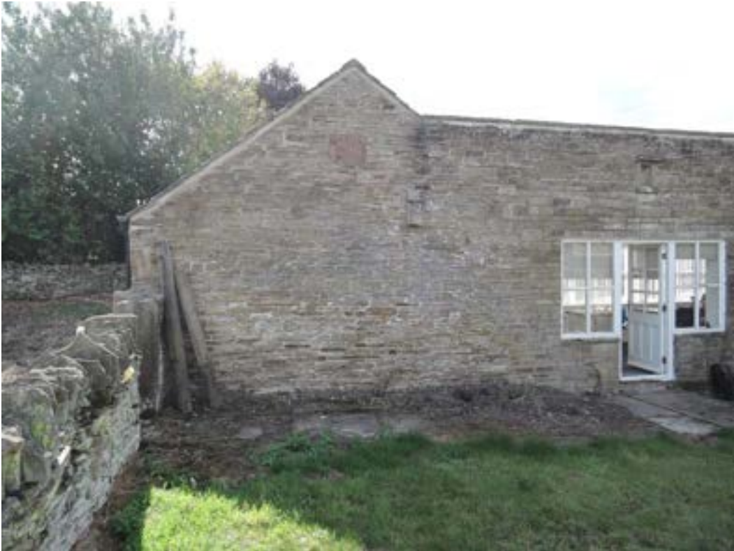
Gable to shed/garage in good order
