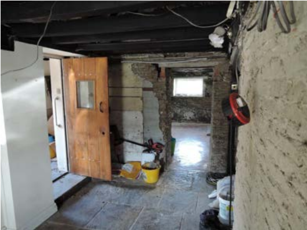
Hallway. Joists over to be replaced in new first floor works
