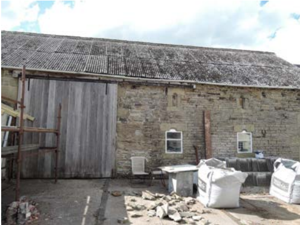
East wall of large barn facing courtyard
