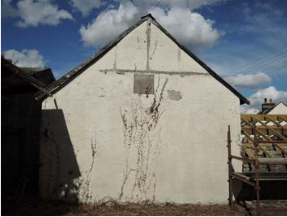
South gable large barn
