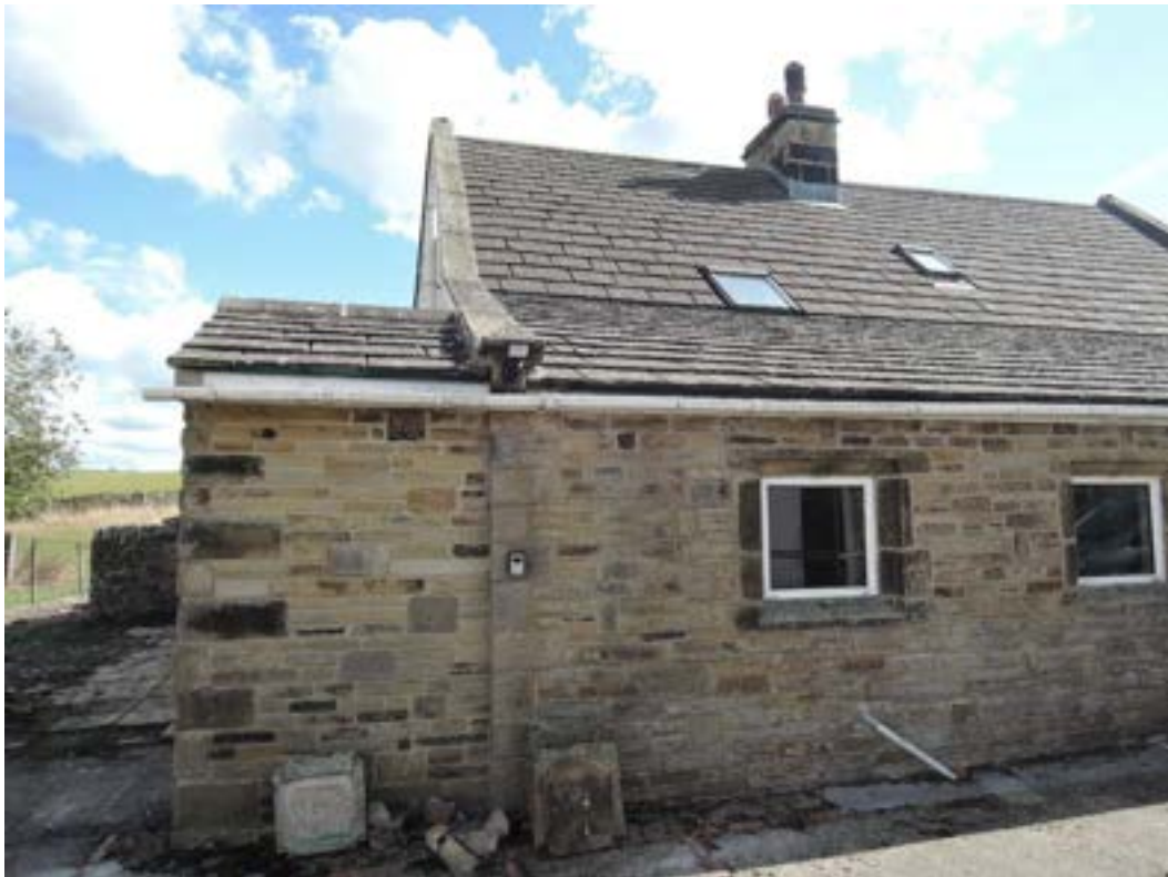
Farmyard side, single storey extension.
