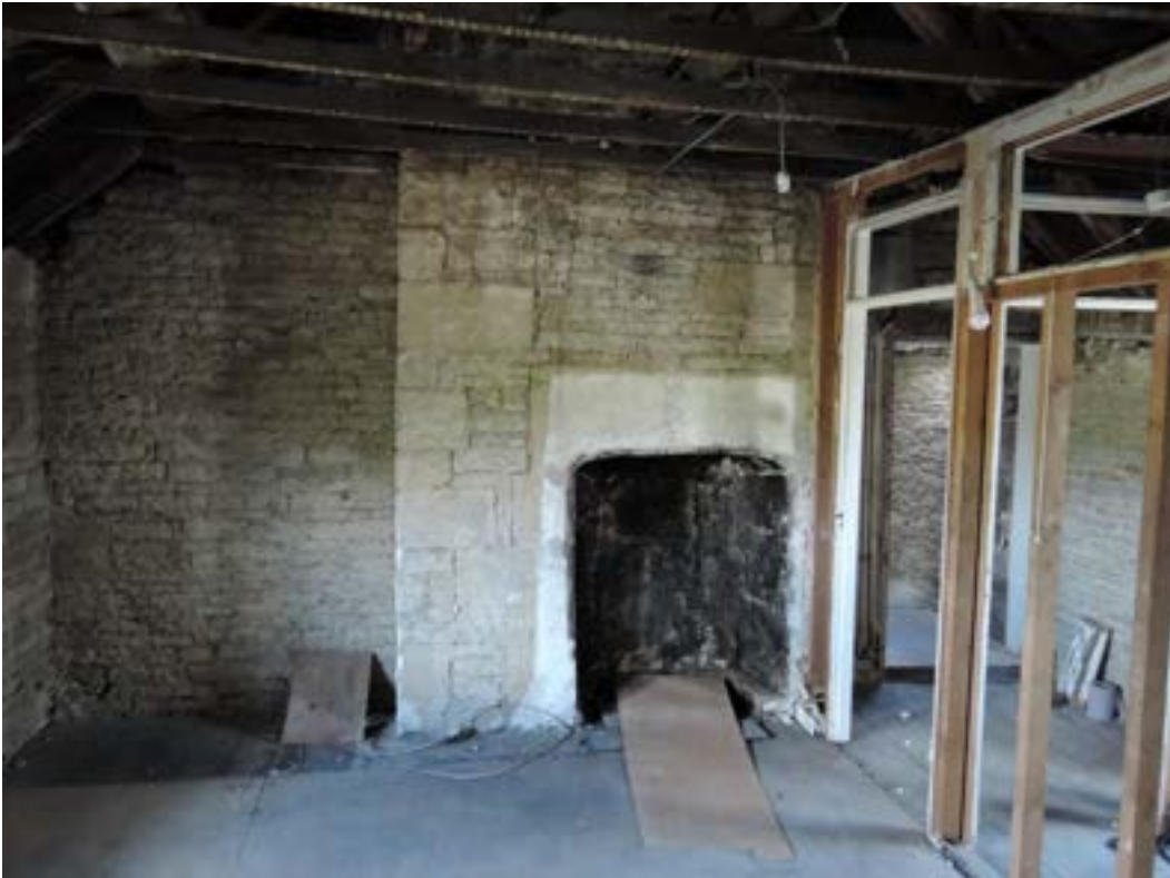
Fireplace in bedroom party wall. Good
