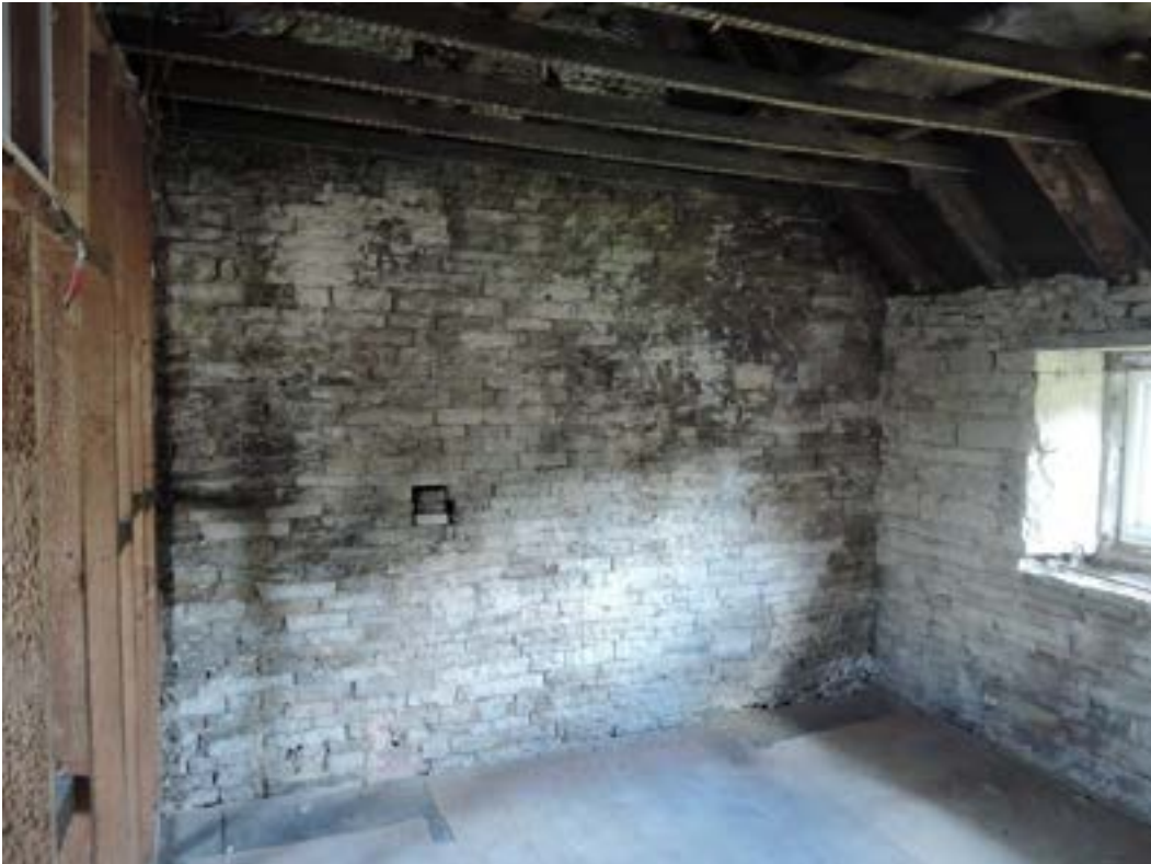
Northeast bedroom gable end. Good.
