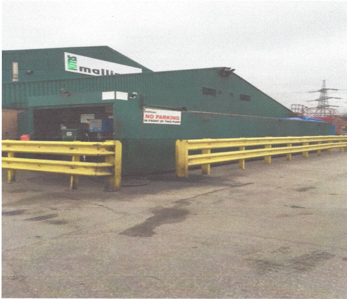
Fig 4 – Ken Mallinson Ltd fuel tank that requires moving to another suitable location
