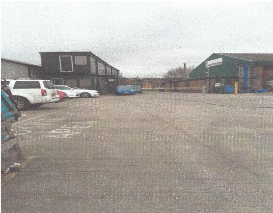
Fig 2 – Ken Mallinson Ltd showing temporary two storey offices
