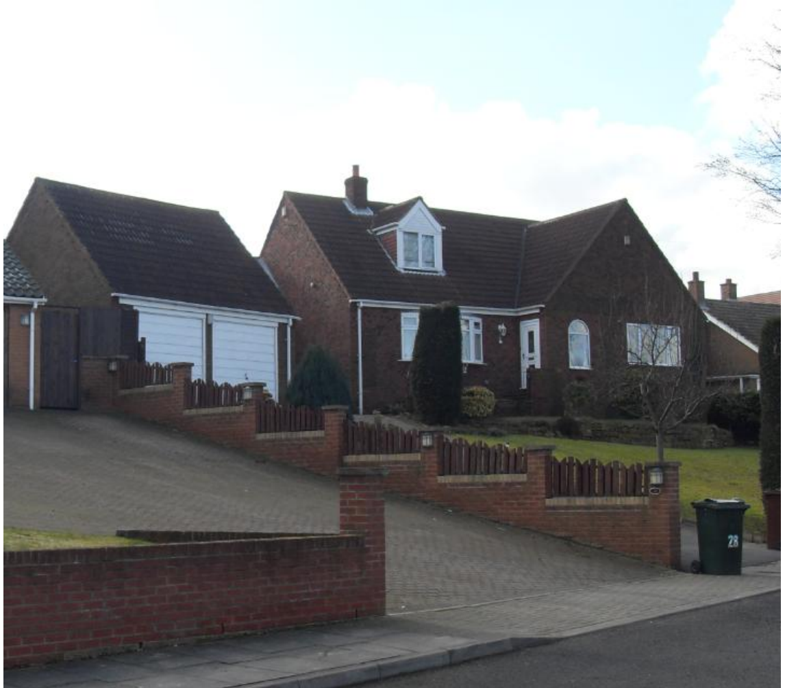
Existing Dwelling Viewed From Melvinia Crescent
