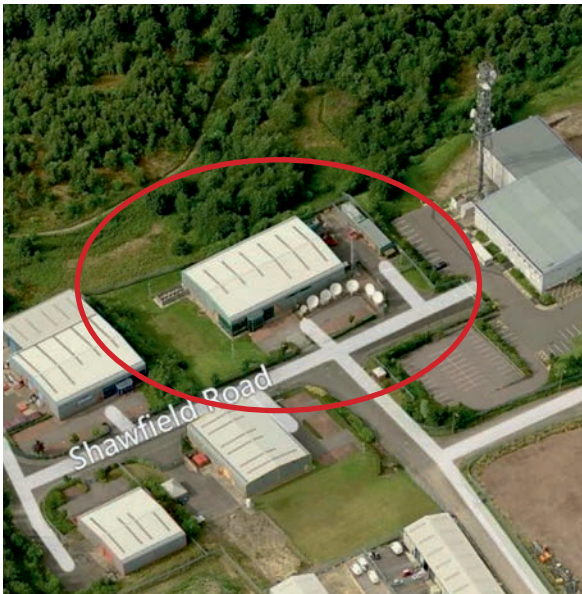
Figure 3. Aerial view of the Virgin Media premises looking from the south.
