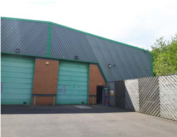
Figure 7. View of the North East elevation, showing the location of the louvres.
