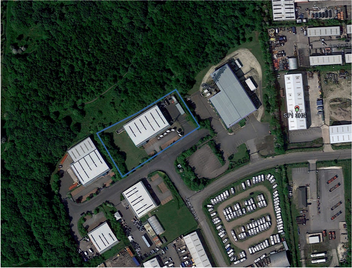
Figure 2. The aerial photograph identifies the Virgin Media site boundary.
