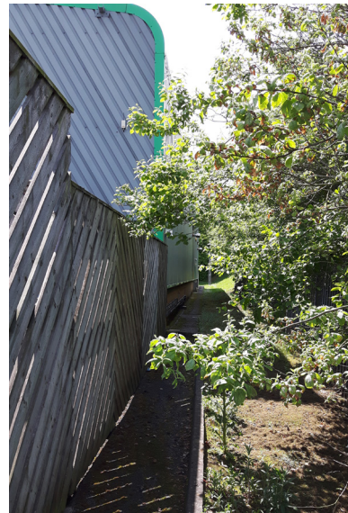
Figure 8. View of the North West elevation, showing the location of the louvres.
