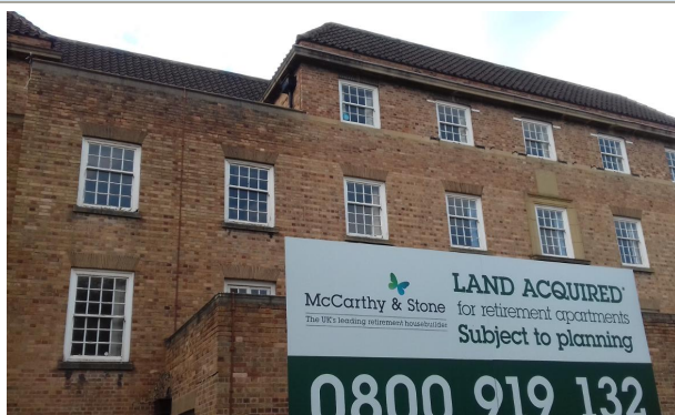
Plate 5. Southern elevation of section 1C, facing north.
