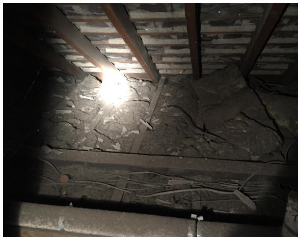
Plate 11. Loft void L2. Example of the dust and debris found within all surveyed loft voids.
