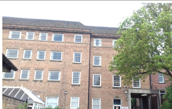
Plate 4. Northern elevation of section 1C, facing south.
