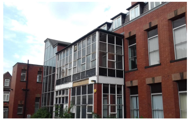
Plate 8. Western elevation of section 1E.
