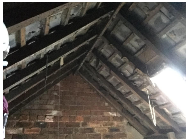
Plate 12. Skylight recorded on the southern end of loft void L3, with a brick wall separating this compartment from the northern end of L3.
