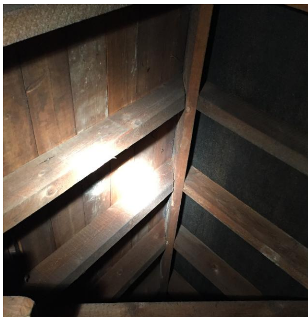
Plate 13. Non-breathable membrane (bitumen felt) and wooden sarking found in loft voids L8 and L9.
