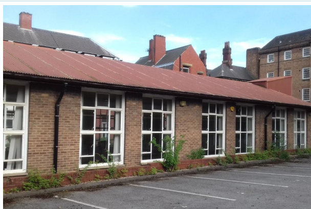
Plate 1. Section 1A, facing southeast
