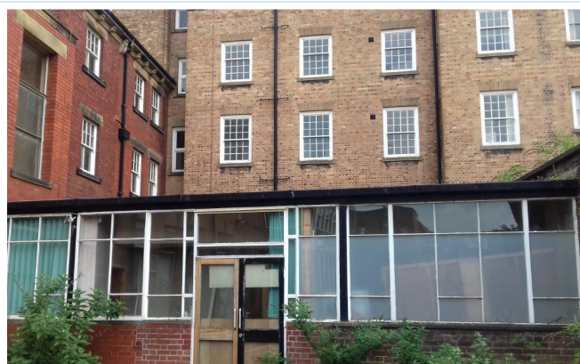
Plate 2. Section 1B, facing south from the central courtyard.
