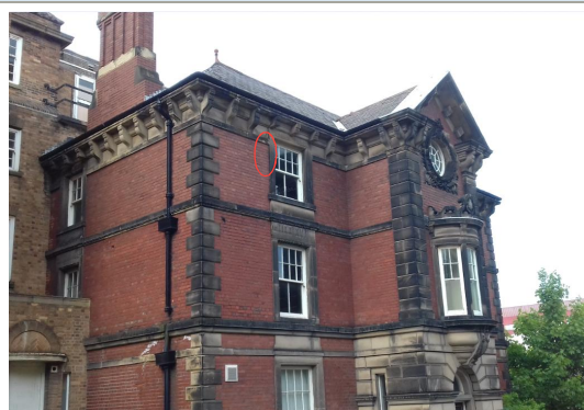
Plate 6. Southern elevation of section 1D, Facing northeast and location of Roost 1D-R4
