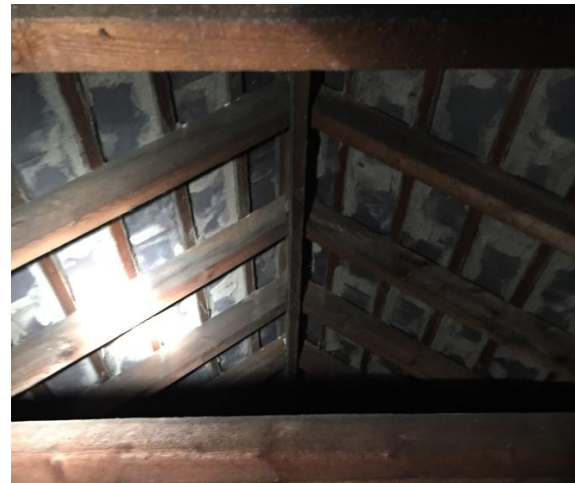
Plate 10. Loft void L1. Example of roofing structure found within the majority of surveyed loft voids (with the exception of L8 and L9).
