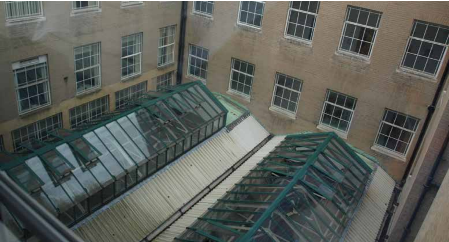
ABOVE: Central light-well, facing north-west.
