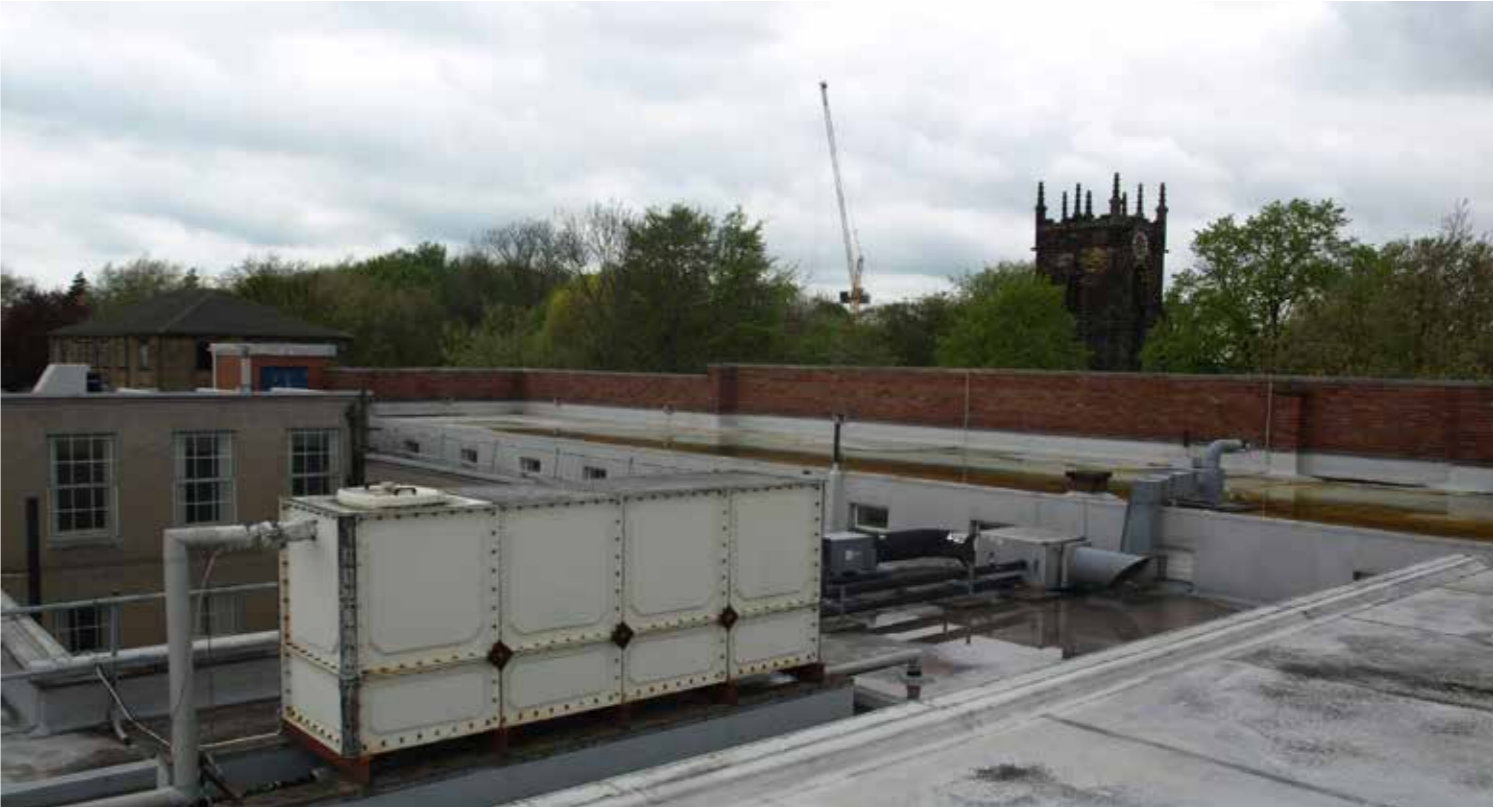
ABOVE: Upper roof level, facing south-east.
