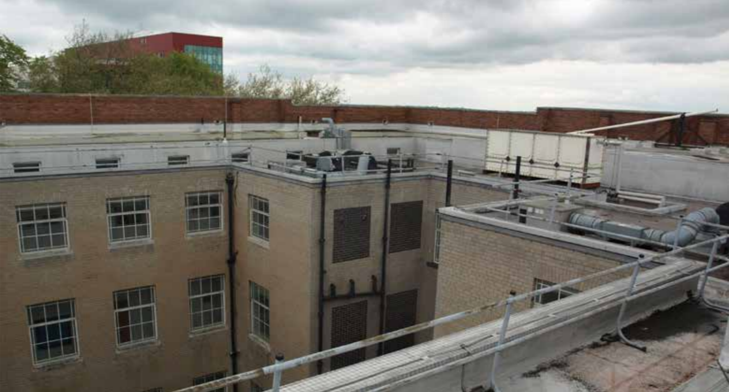
ABOVE: Upper roof level, facing north-east.
