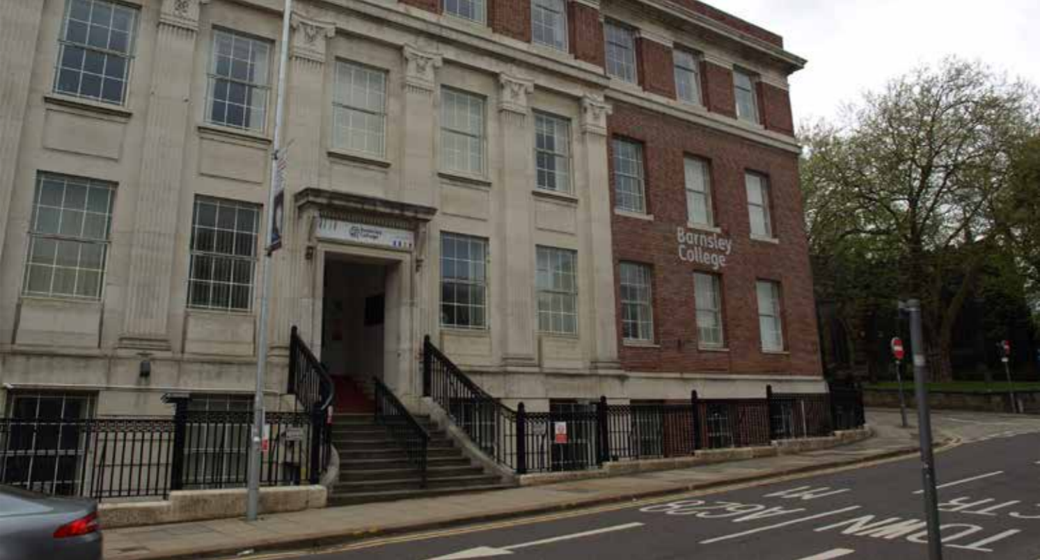
ABOVE: Building main eastern entrance, facing west.
