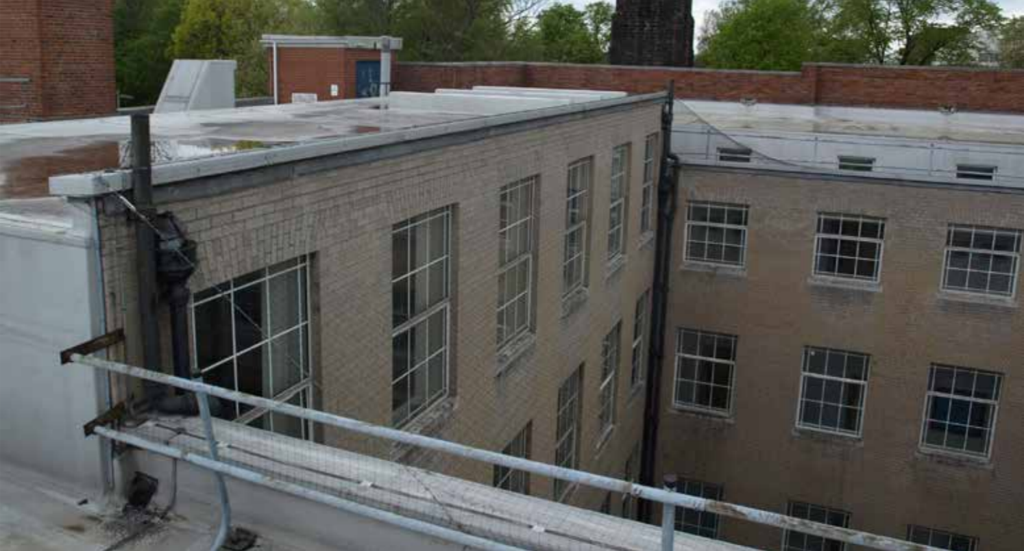
ABOVE: Upper roof level, facing north-west.
