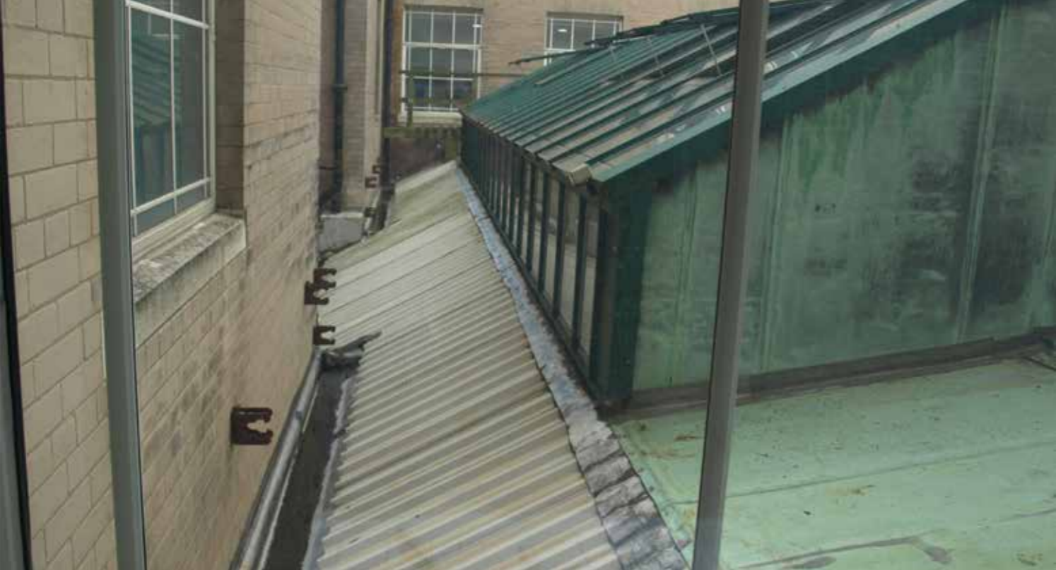
ABOVE: Central light-well, facing south.
