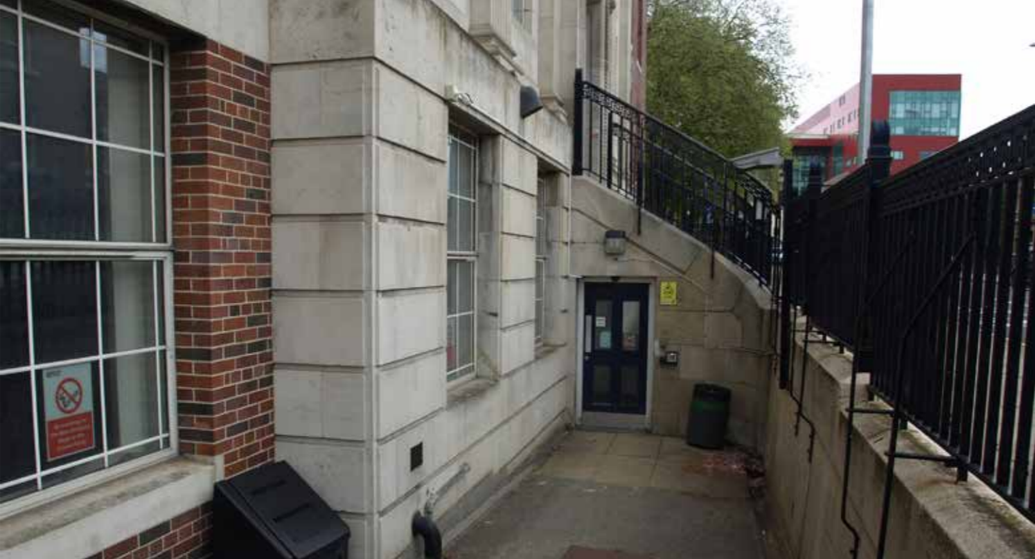
ABOVE: Arch link bridge of building main eastern entrance, taken at Level 01 facing north.
