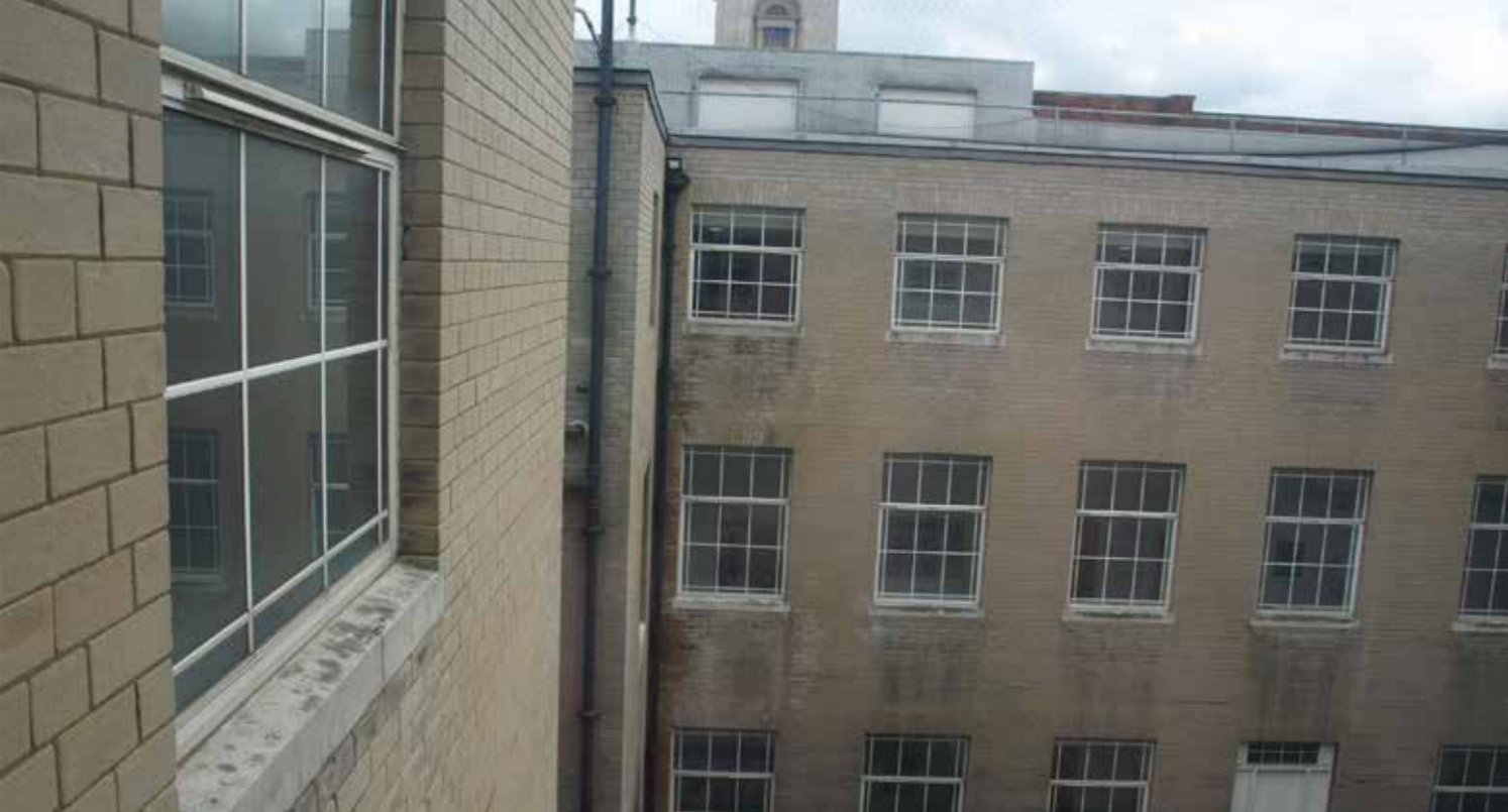
ABOVE: Central light-well, facing south
