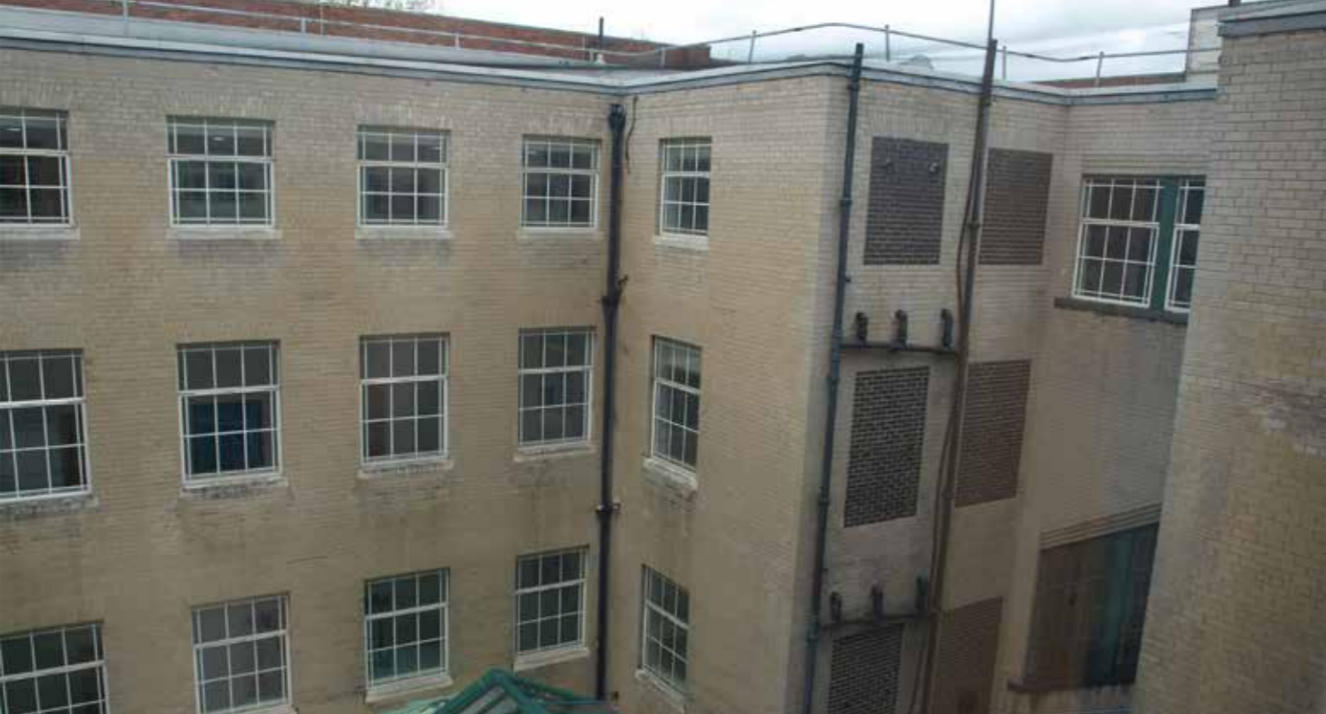
ABOVE: Central light-well, facing north-east.
