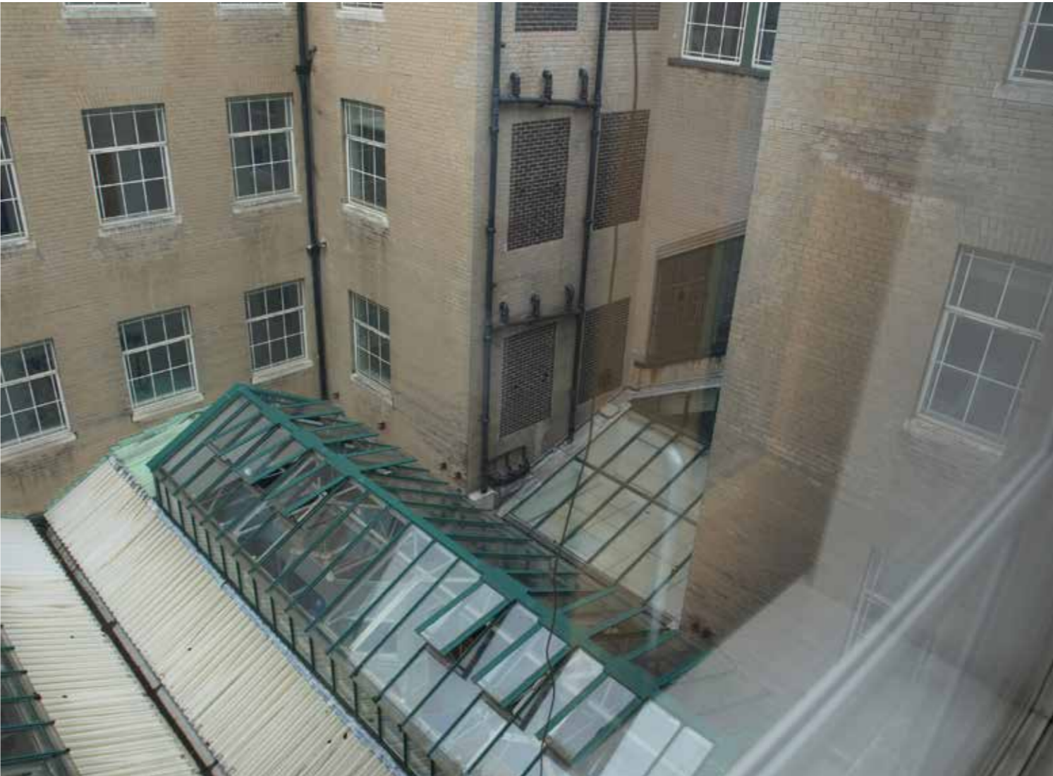
ABOVE: Central light-well, facing north-east.
