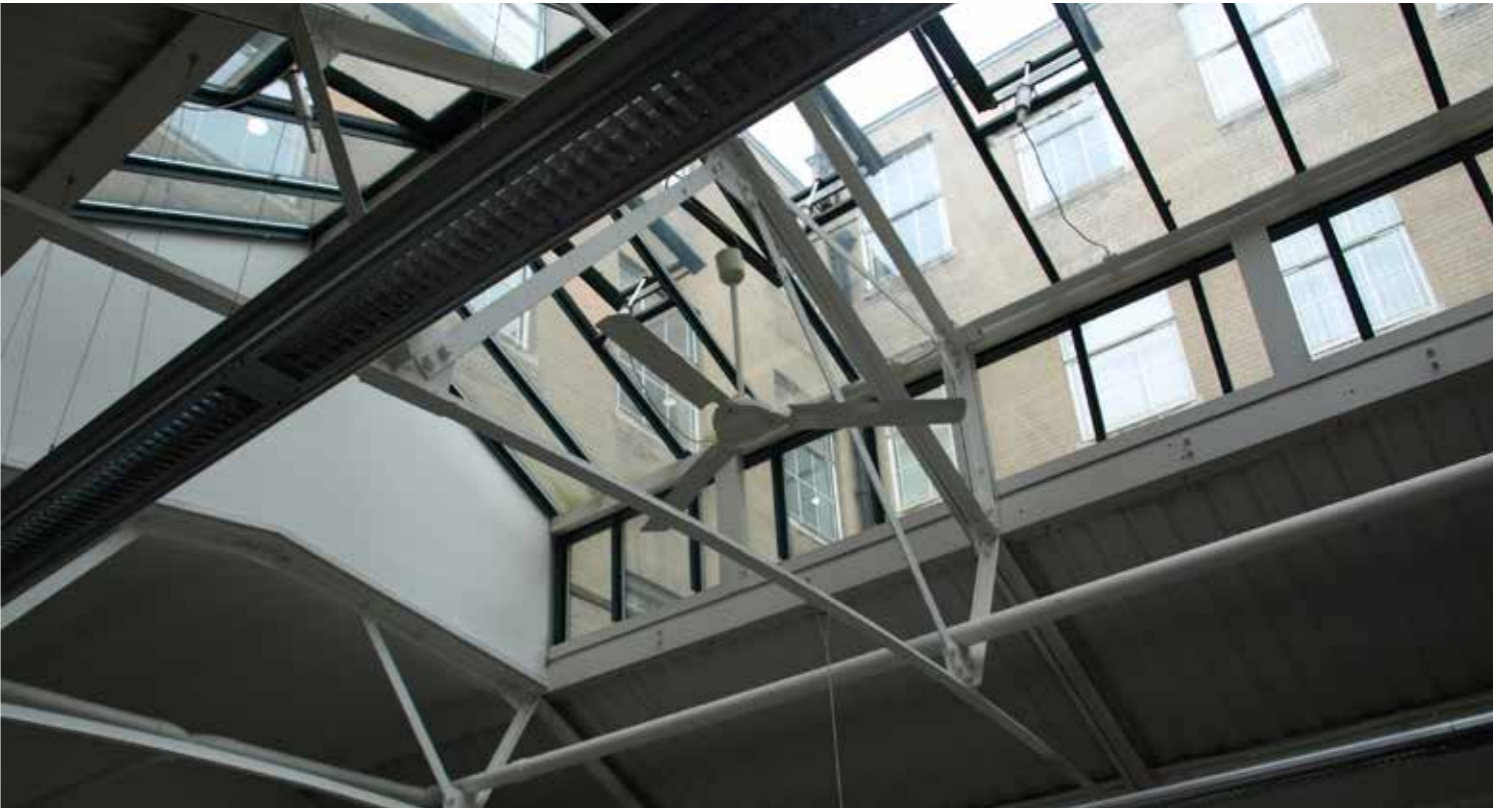
ABOVE: Level 01 Library space, facing south-west.
