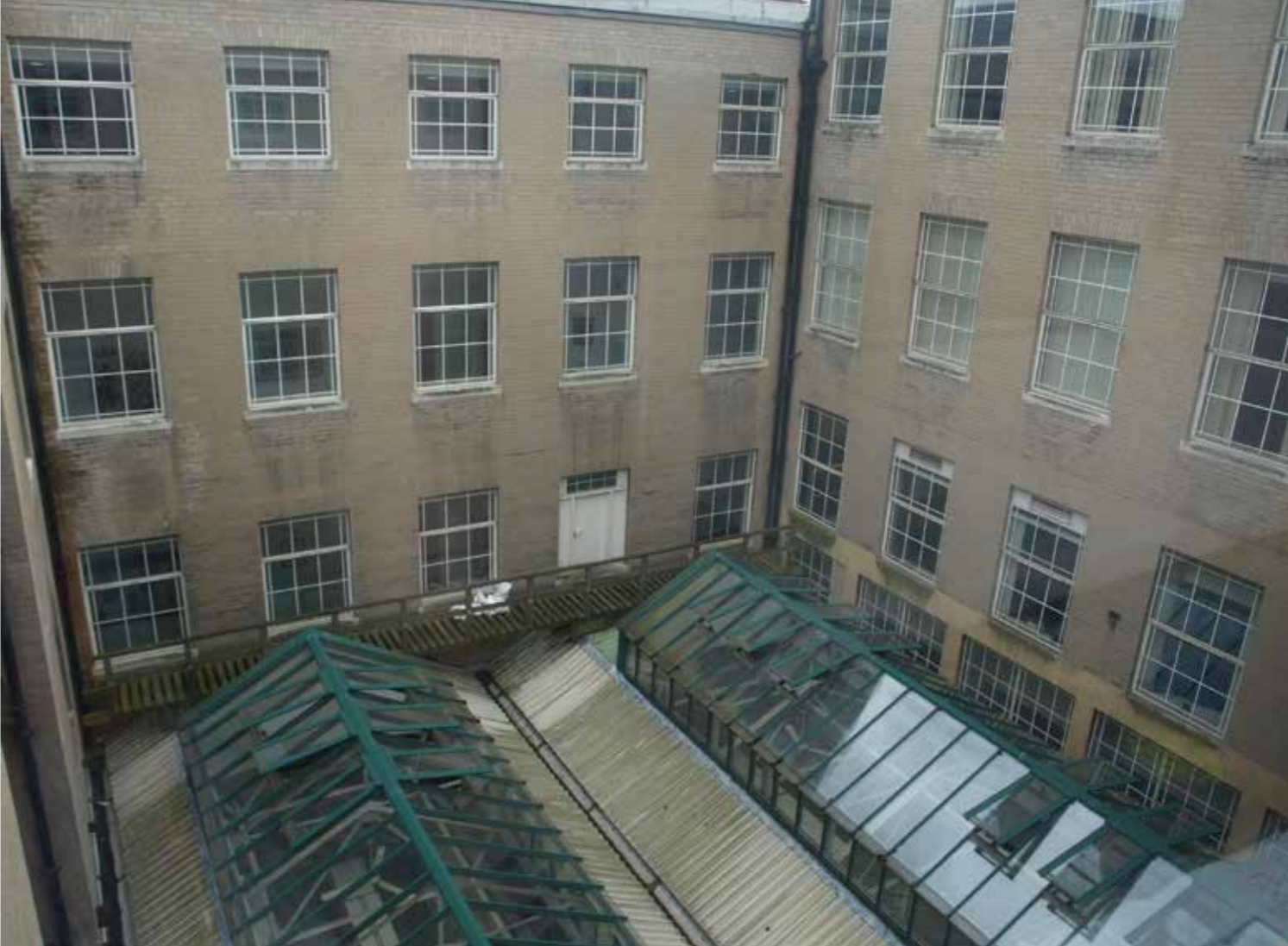
ABOVE: Central light-well, facing south-west.
