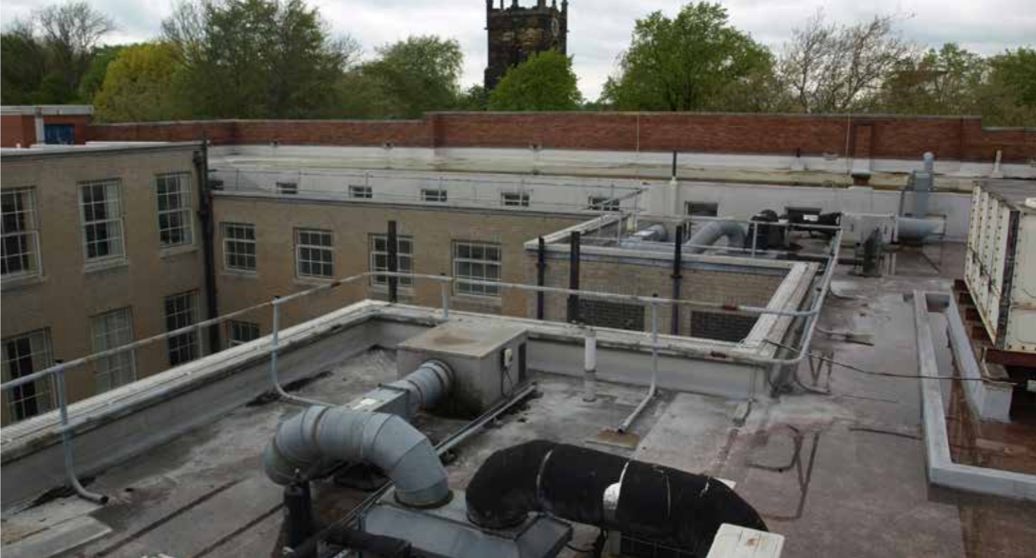
ABOVE: Upper roof level, facing north-west.
