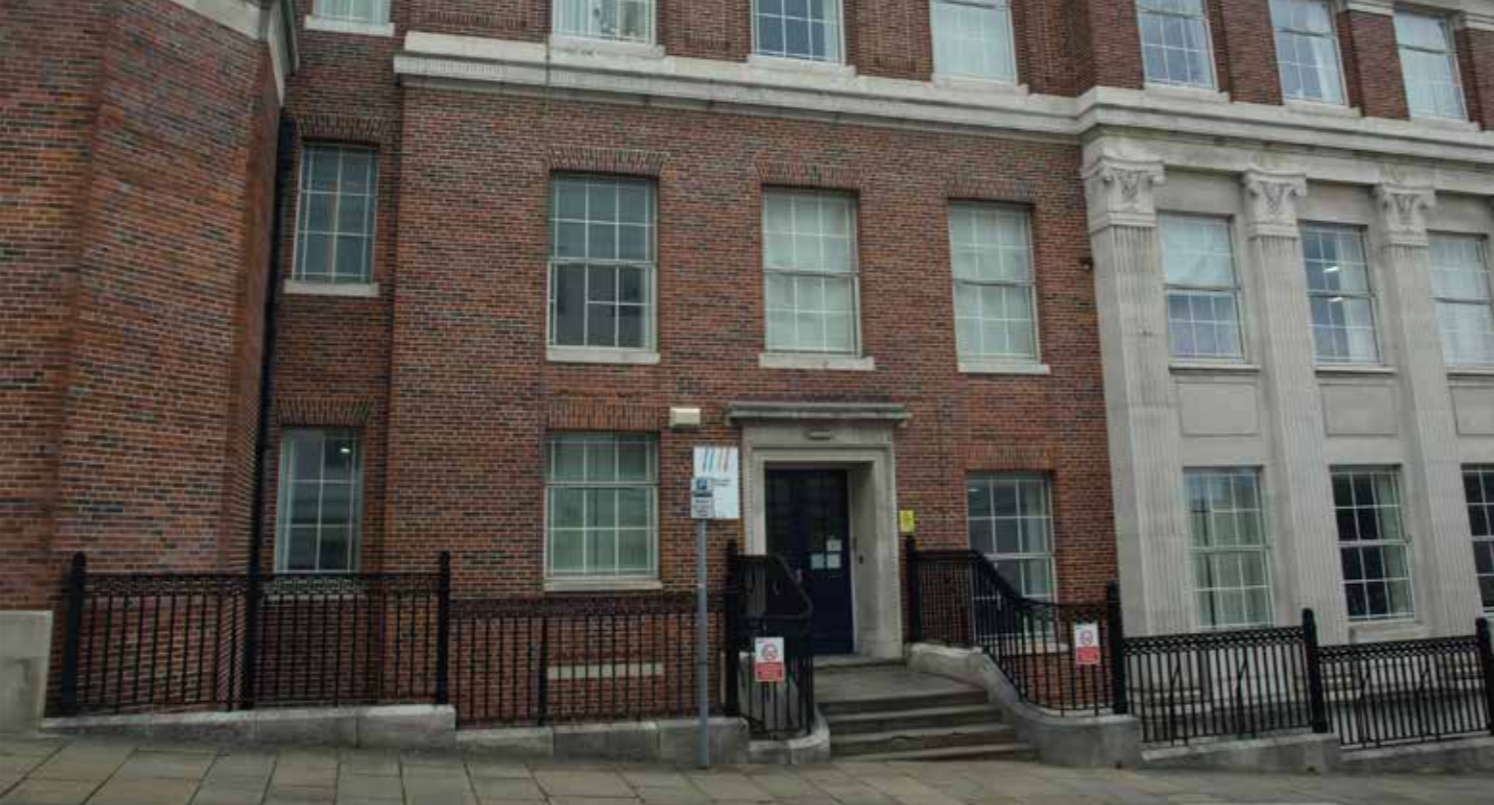
ABOVE: Building side southern entrance, facing north.
