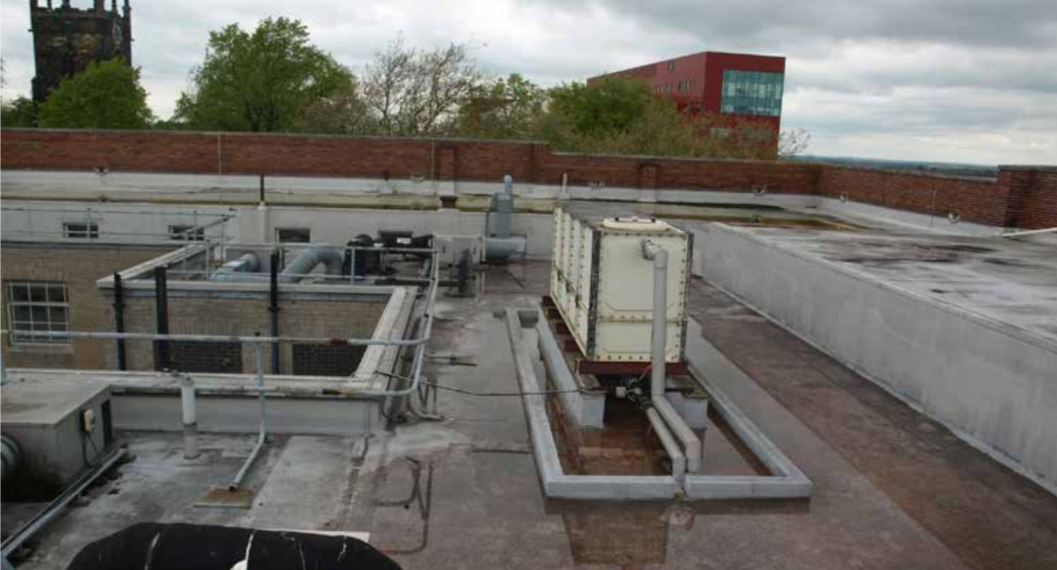
ABOVE: Upper roof level, facing north.
