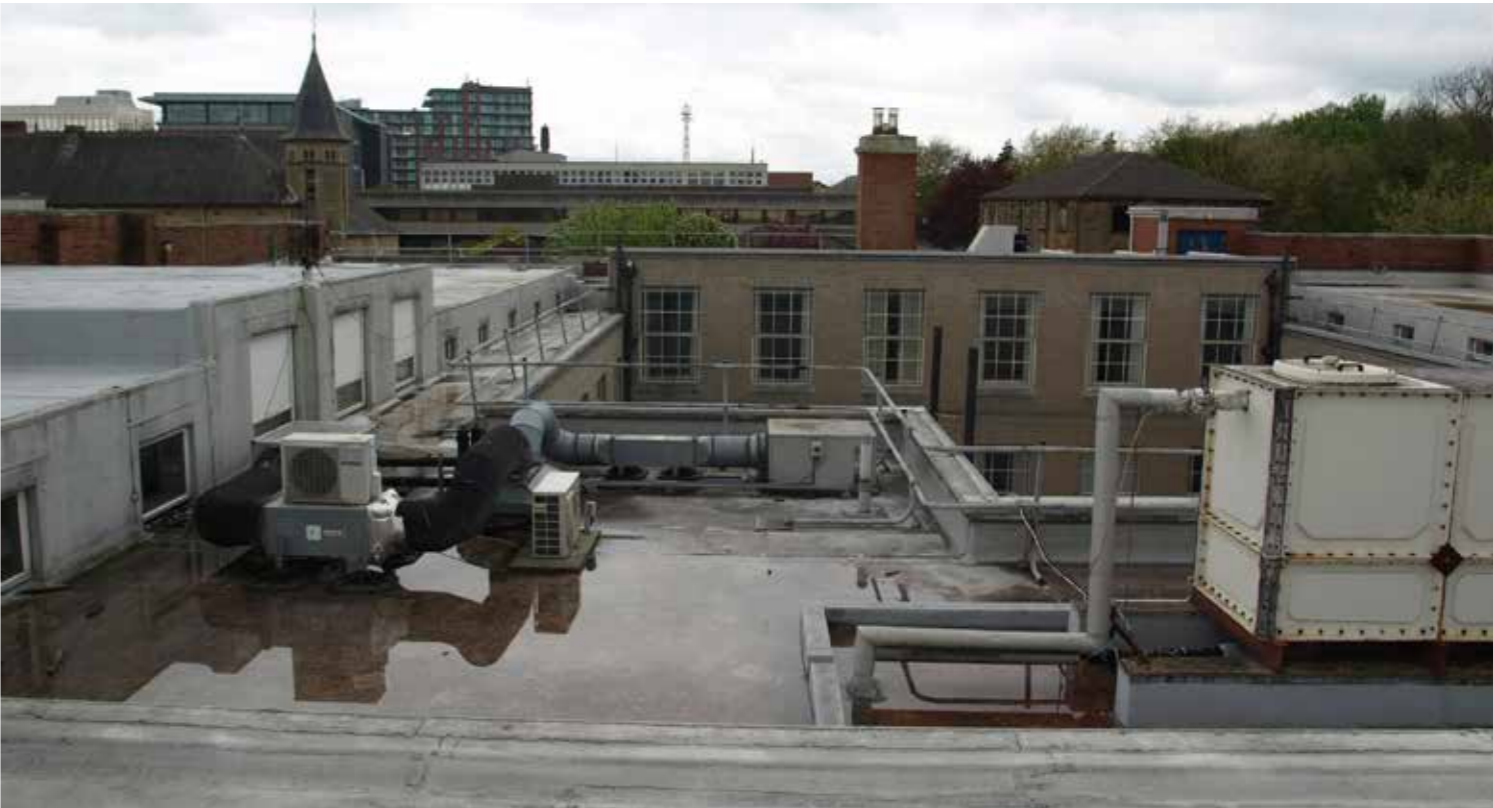
ABOVE: Upper roof level, facing west.
