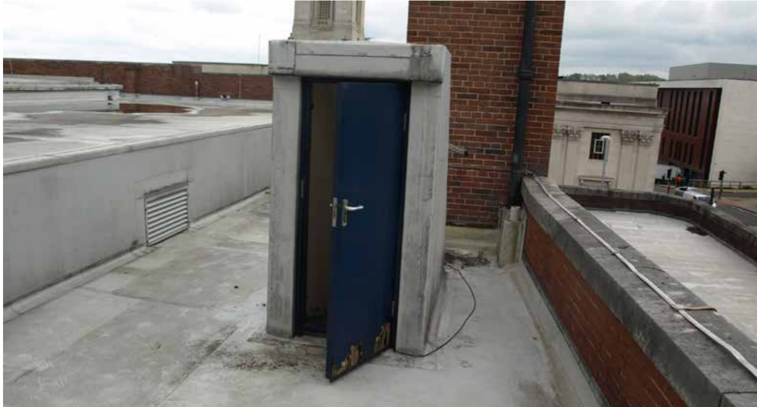
ABOVE: Upper roof level access door, facing south.
