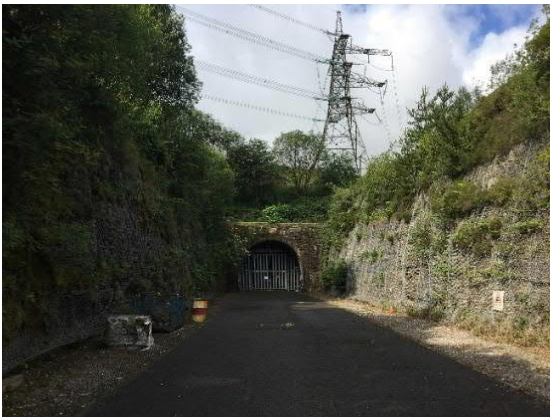
Photo 4: General view of south culvert
