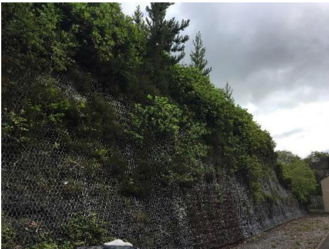
Photo 5: R5 extending to end of raised area.
