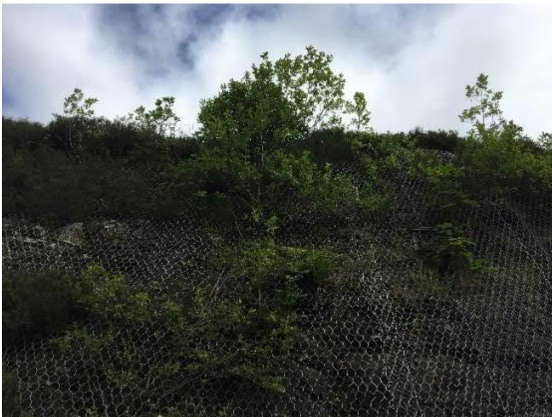
Photo 3: R3 at topmost part of culvert wall.
