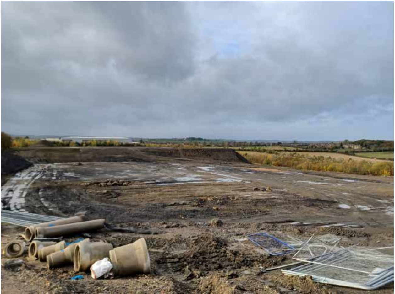
Photograph No 1: Taken on 12 November 2021 – Mound 1 Surcharge in background and Mound 2 plateau in foreground.
