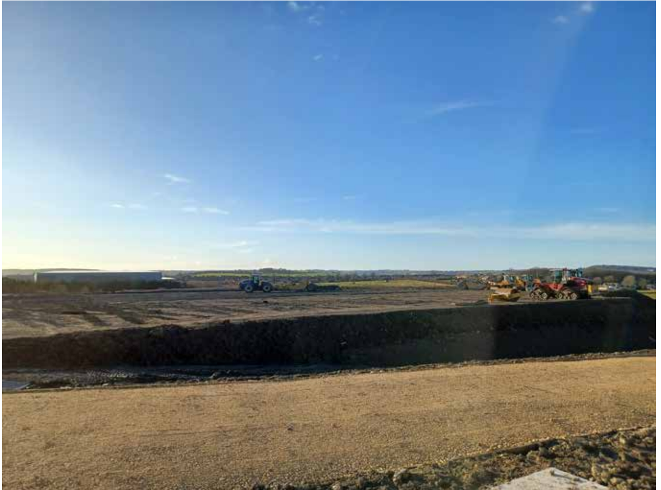
Photograph No 5: Photograph taken on 20 January 2022 – Progress of Mound 2 Surcharge.
