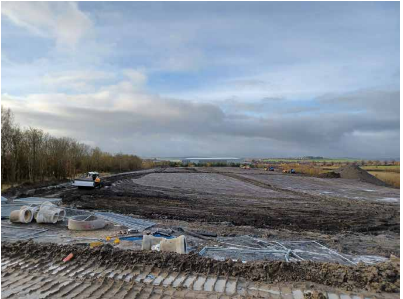
Photograph No 4: Photograph taken on 9 December 2021 – Progress of surcharge material movement from Mound 1 to Mound 2 Position.
