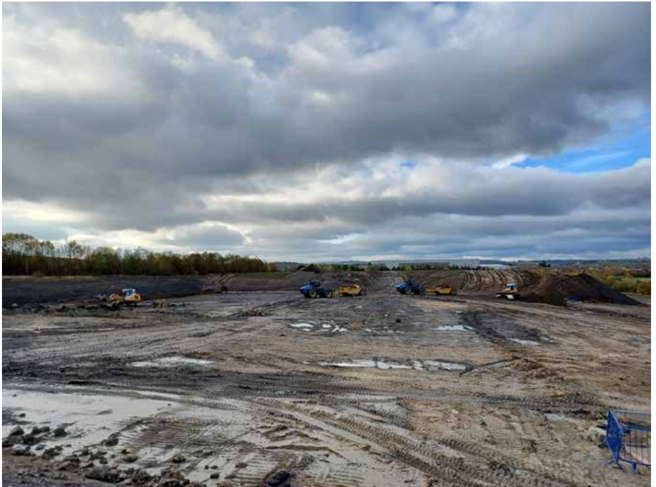
Photograph No 3: Photograph taken on 24 November 2021 – Beginning of surcharge material movement from Mound 1 to Mound 2 position.
