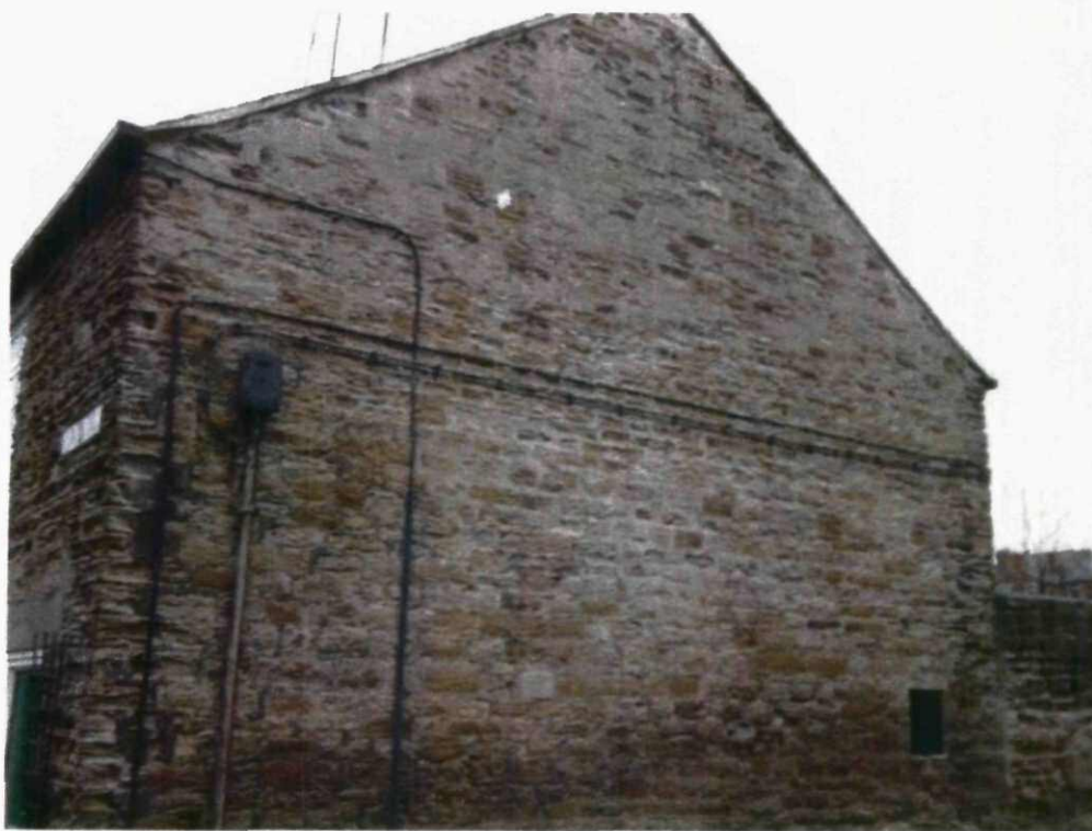
Photo 1- Gable Wall to 1 Old Row
