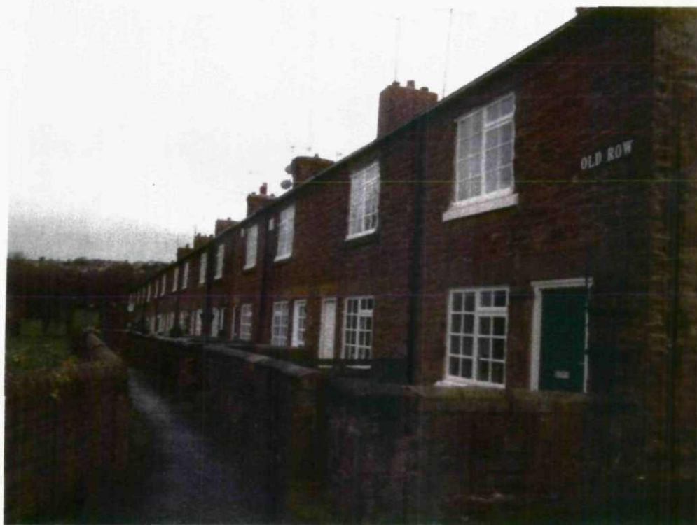
Photo 2- Front Elevation to Old Row from No 1
