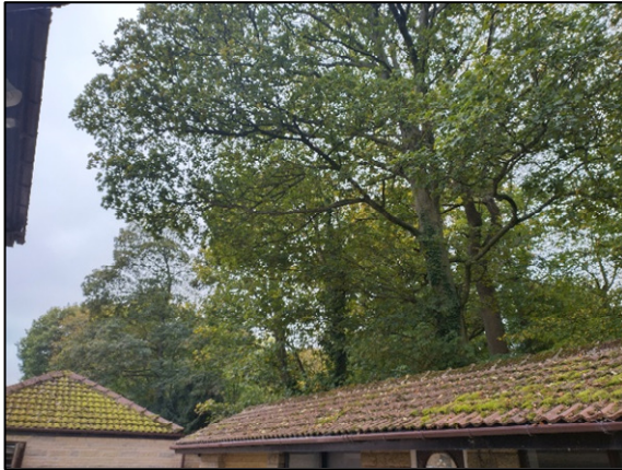
Photo 1: T1, T2, and G8 looking south east
