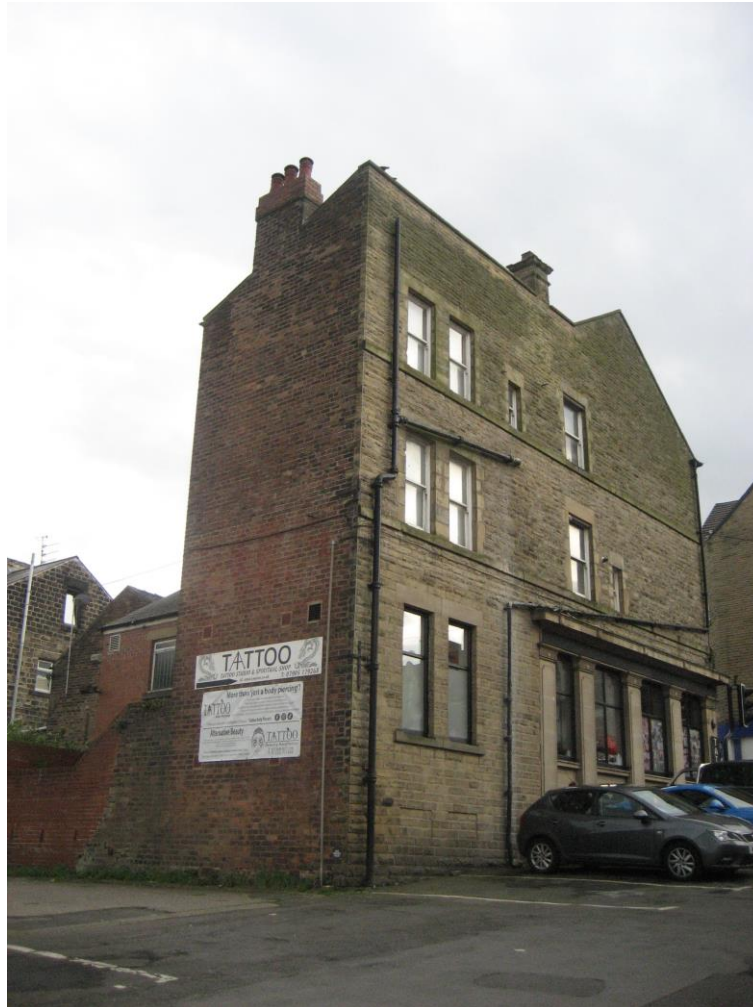
Side/Rear View from North in Car Park.
