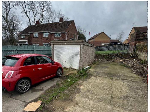
Photo 4: The garage on site.
