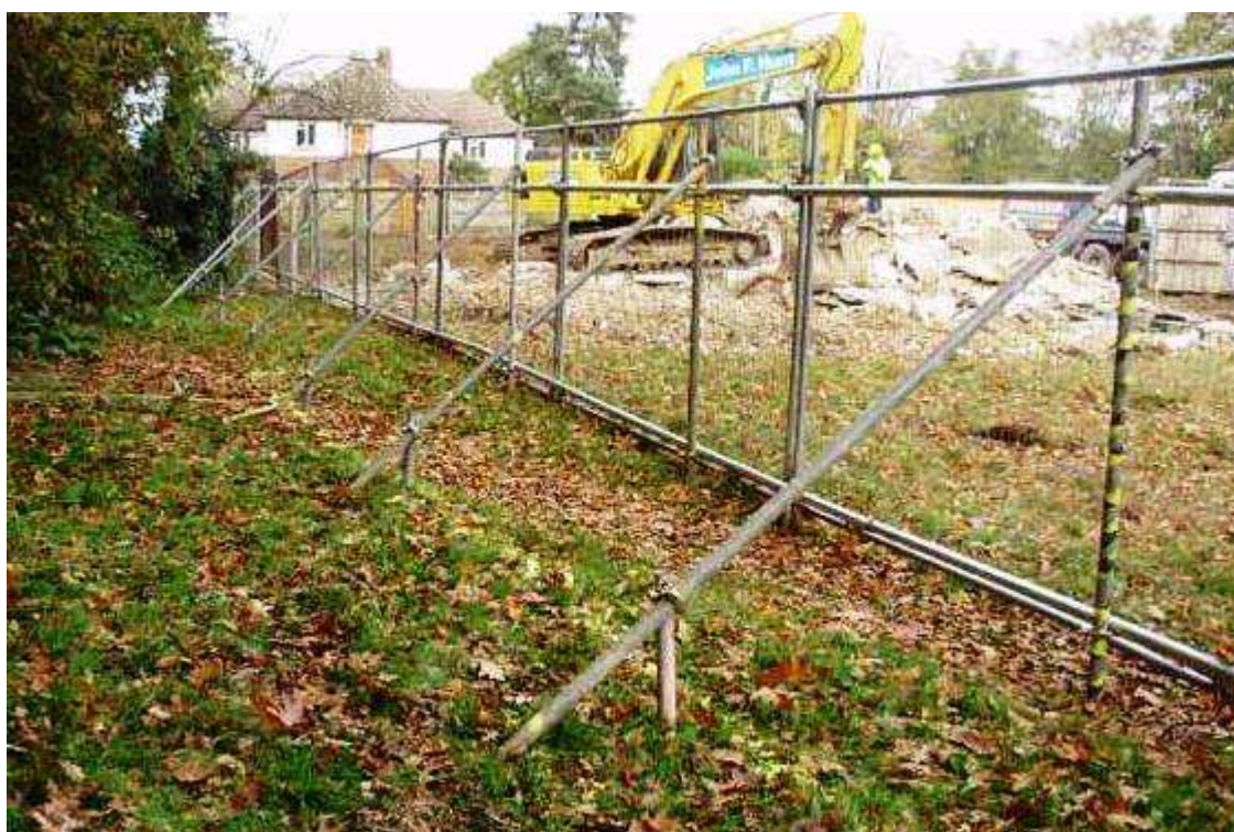
Figure 2: 'Photo of Fencing to BS 5837: 2012'.
