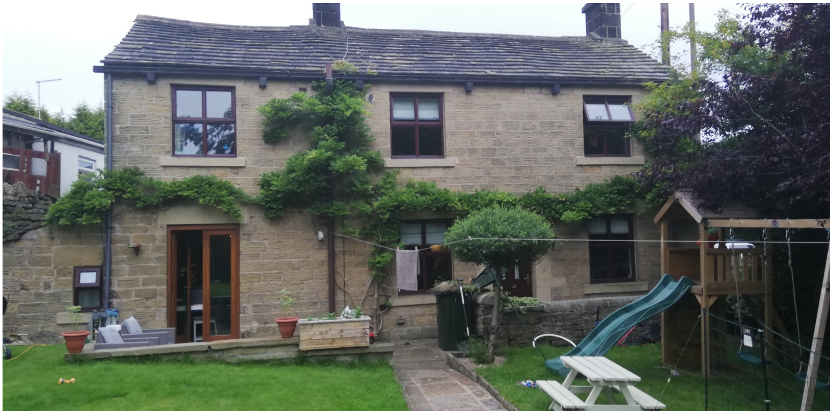
East elevation and garden
