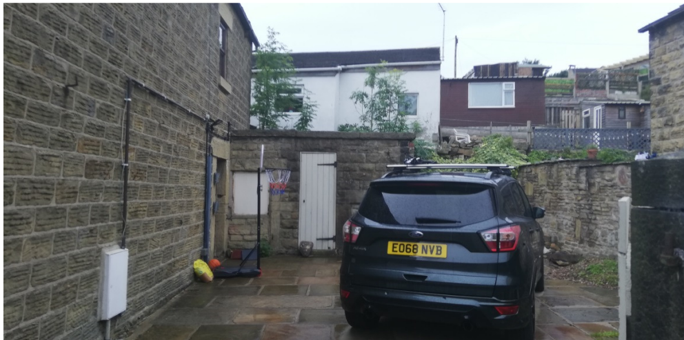
View of the yard, showing a remaining wall of an outbuilding outbuilding
