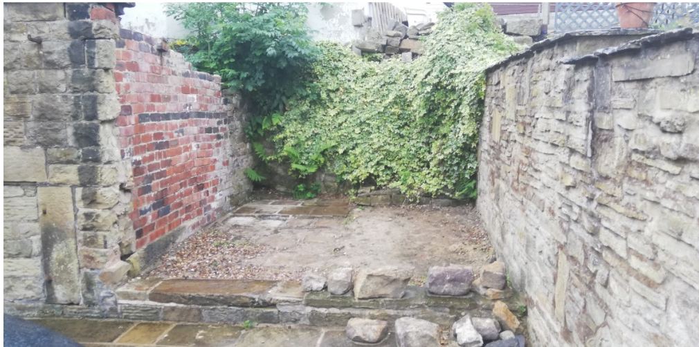
The southern boundary and partly demolished outbuilding from the yard
