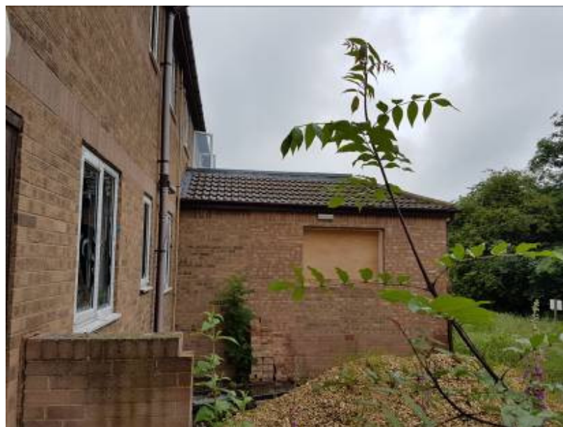
General view of the building & location of soffit gap
