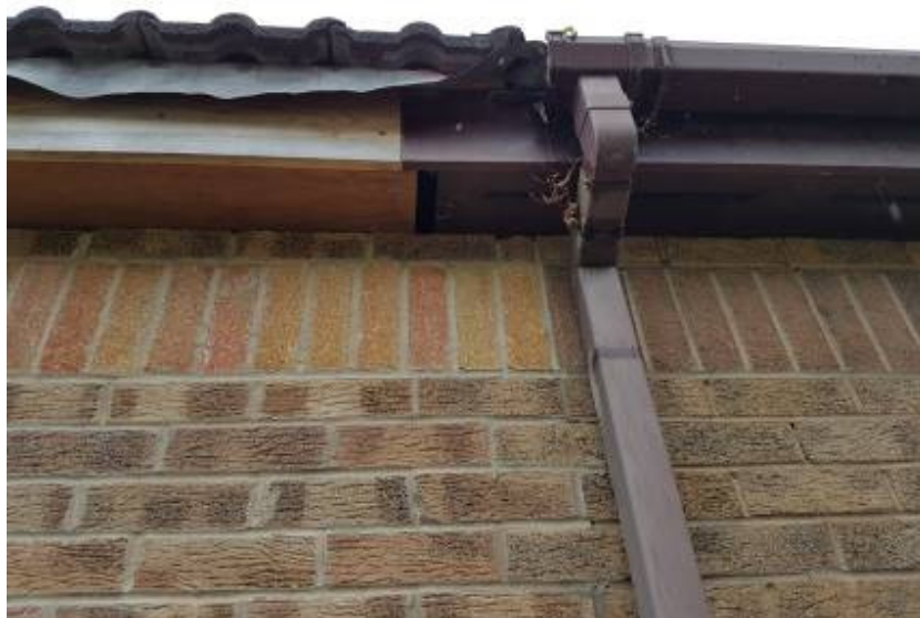
General tight nature of soffits
