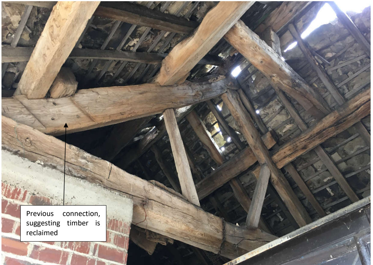
11. Timber Truss in Building 1
