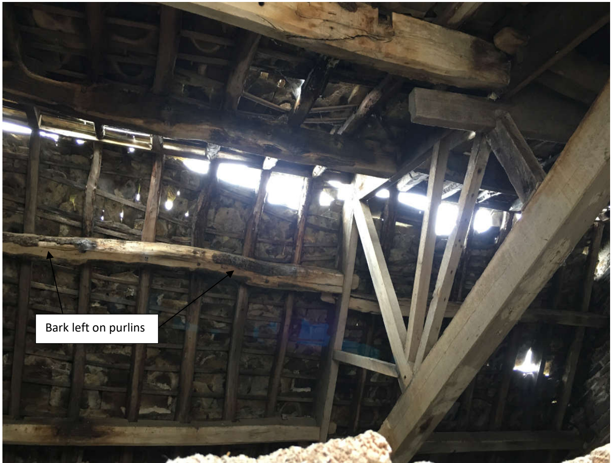
19. Roof Structure to Building 4
