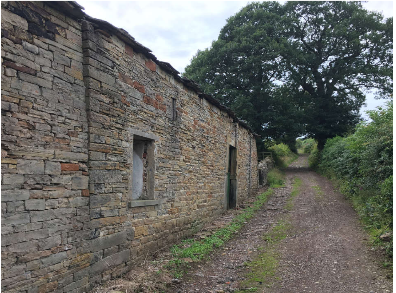
3. West Elevation of Buildings 1 and 2
