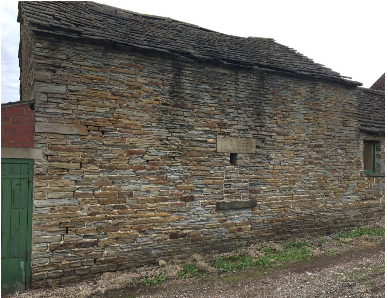
5. West Elevation of Building 4
