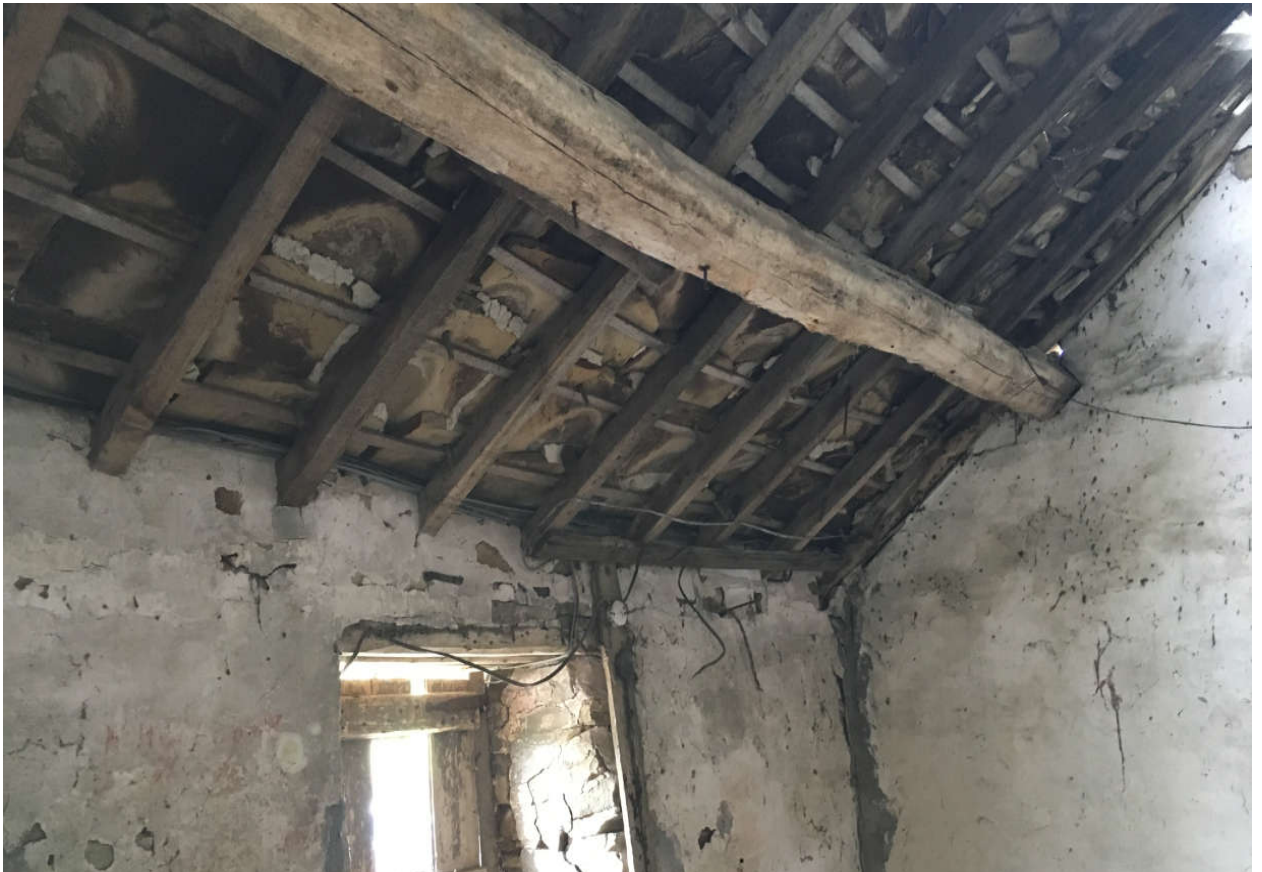
14. Roof Structure to Building 2
