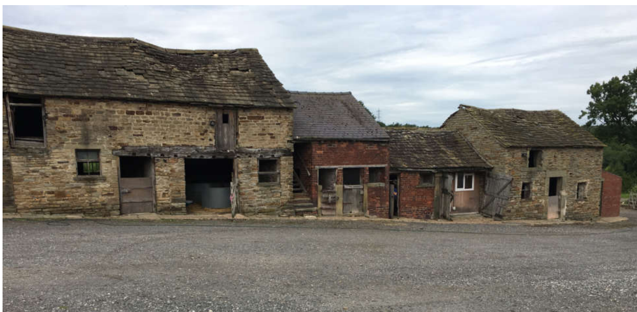
2. East Elevation of Buildings 2, 3, 4 and 5
