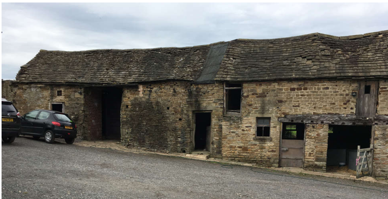
1. East Elevation, Buildings 1, 2 and 3
