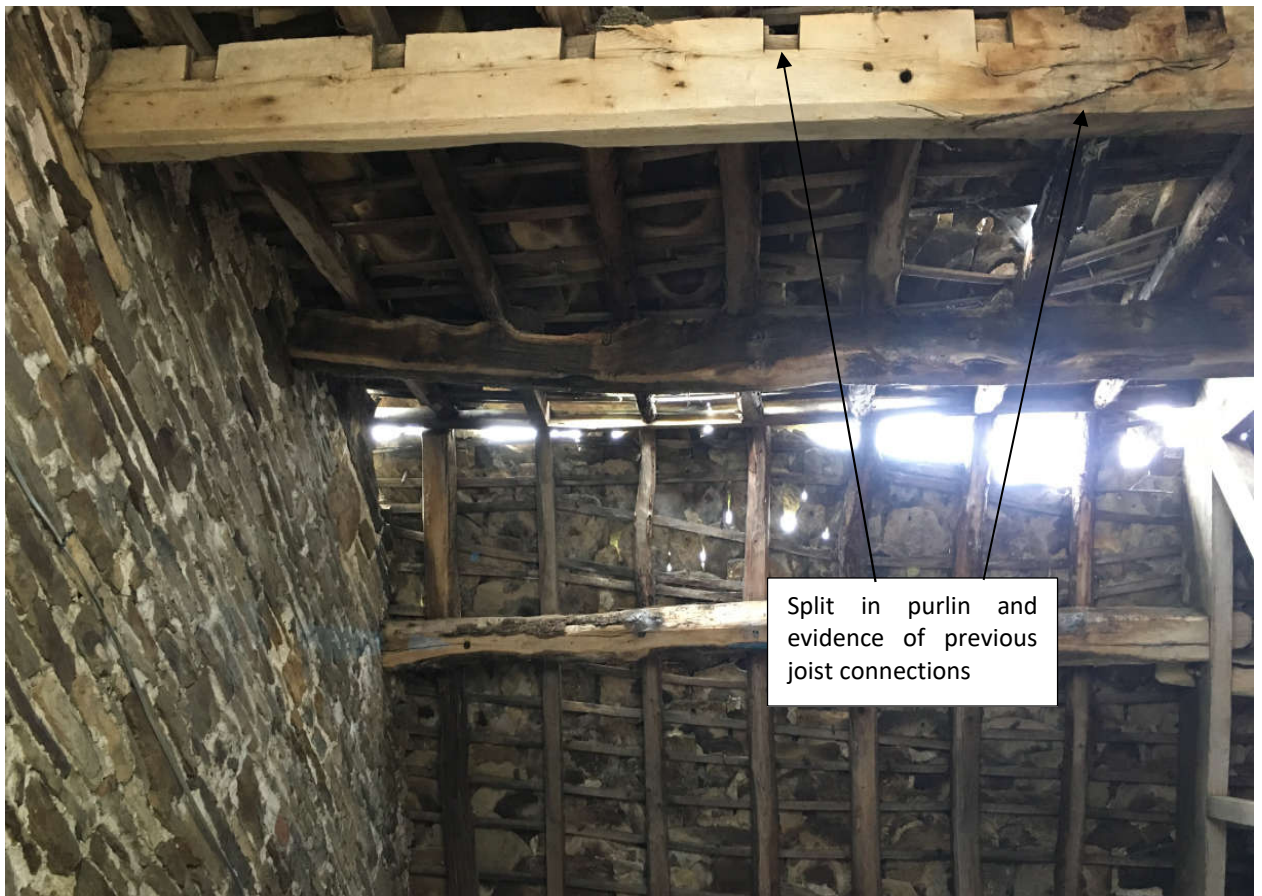
20. Purlins to Building 4
