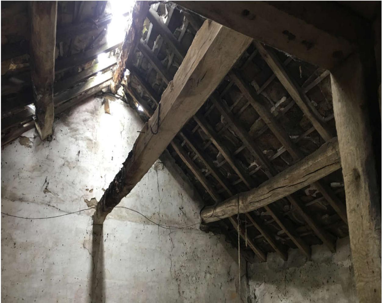
13. Roof Structure to Building 2
