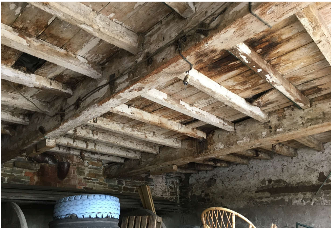
24. Floor Structure to Building 4
