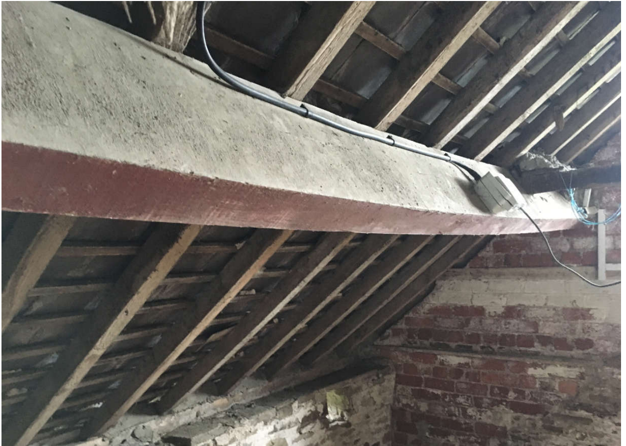
15. Purlin in Building 3 (Two storey part)
