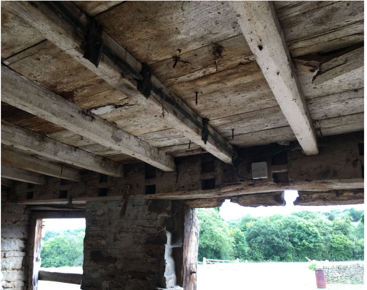
23. Floor Structure to Building 2
