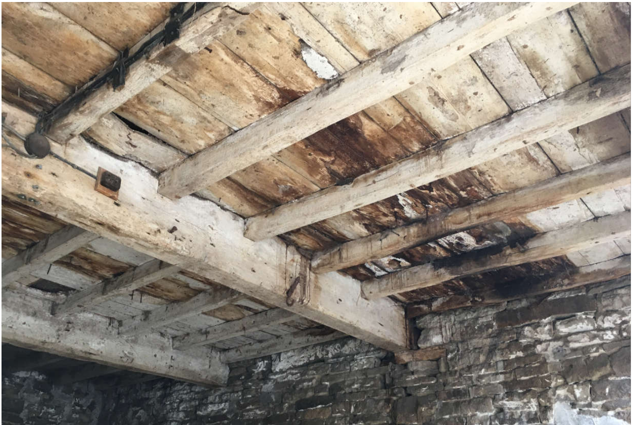
22. Floor Structure to Building 2
