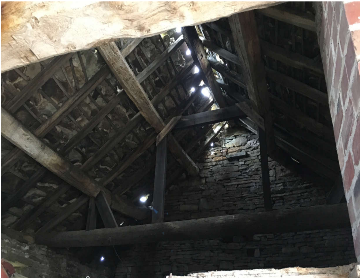
12. Timber Truss in Building 1
