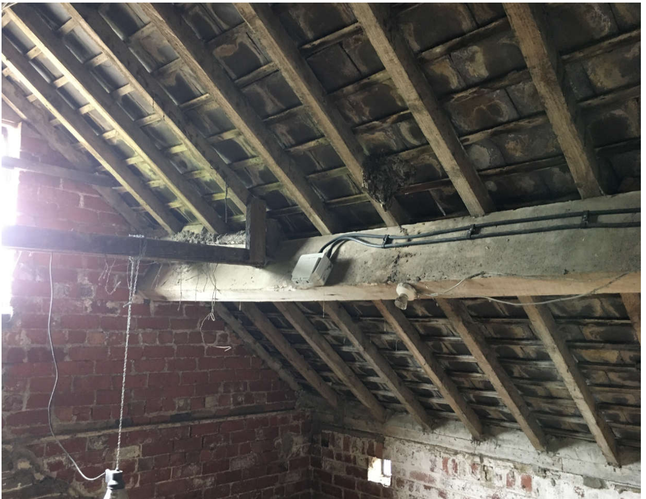
16. Purlin in Building 3 (Two storey part)
