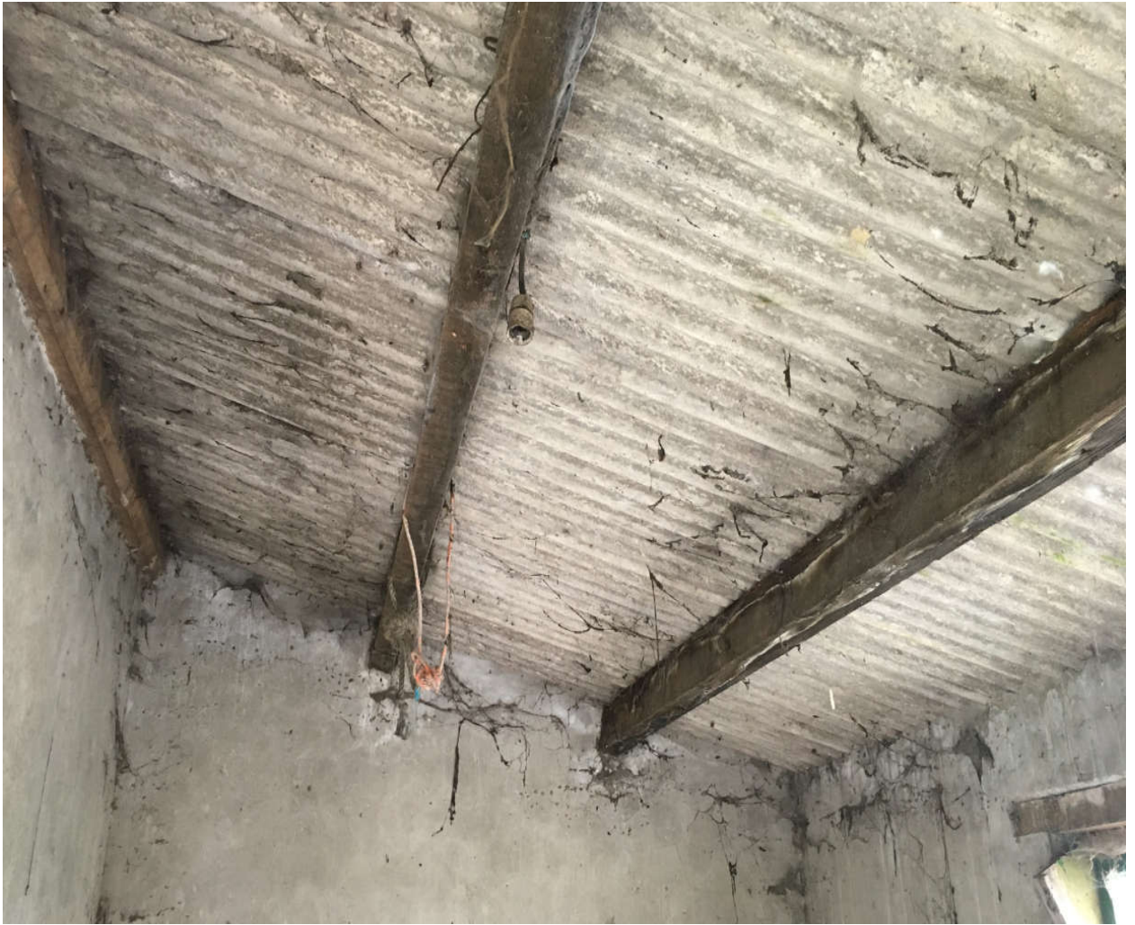
21. Roof Structure to Building 5
