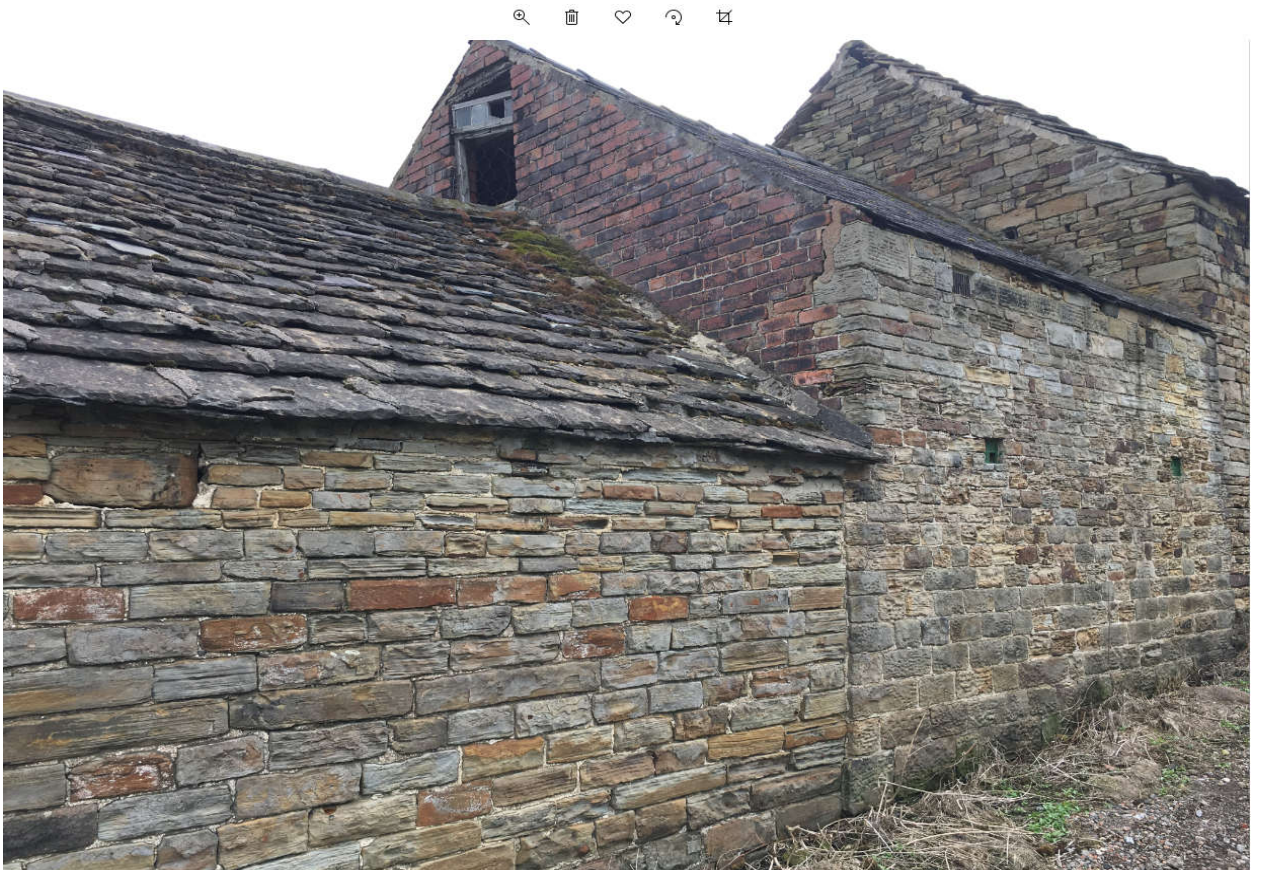
4. West Elevation of Building 3
