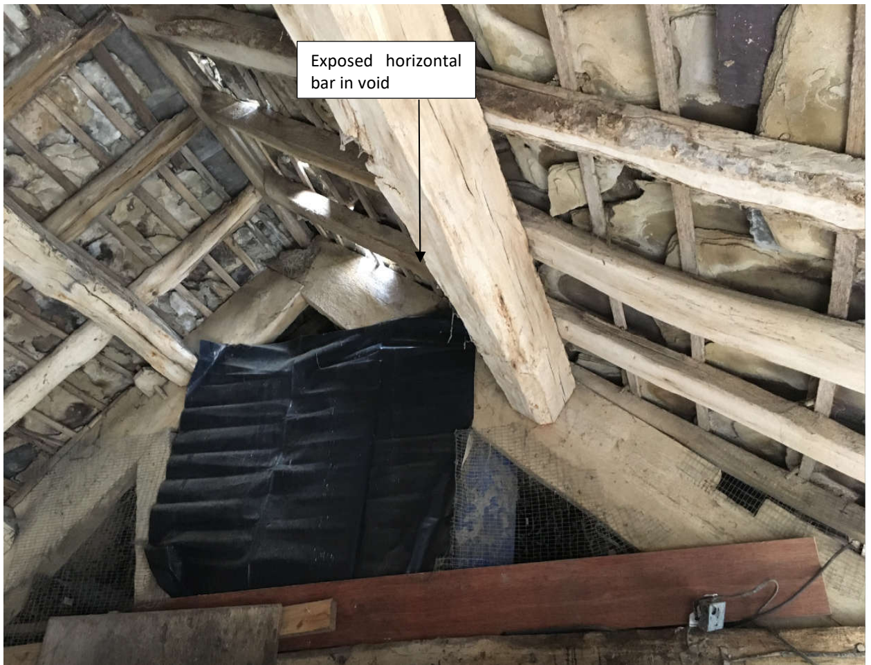
17. Roof Structure to Building 3 (Single storey part)
