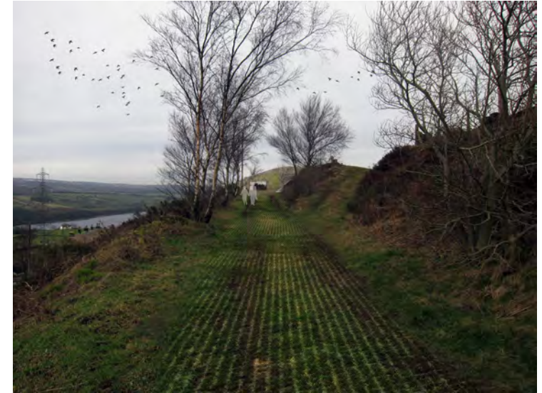
Visualisation of the building from part way along the access track. - even here the building is barely visible.
