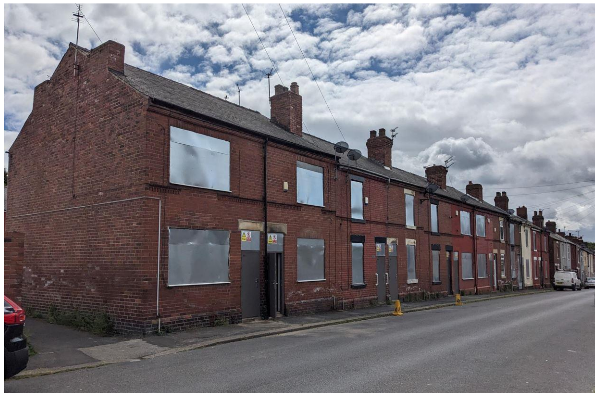
Above: Photo of existing terraced properties proposed for demolition on Co-Operative Street to be replaced by New Build Housing & open space
