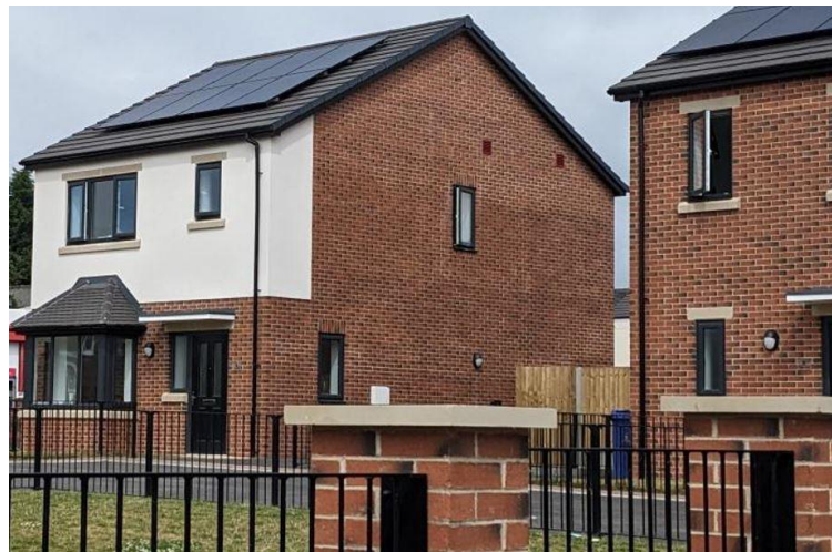
Solar PV panels & associated batteries fitted to Lapwing View dwellings
