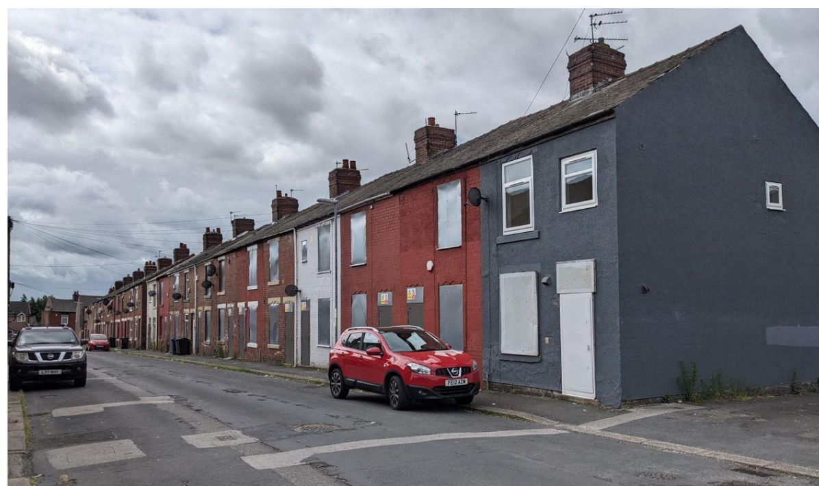
Above: Photo of existing terraced properties proposed for demolition on Victoria Street to be replaced by New Build Housing & open space
