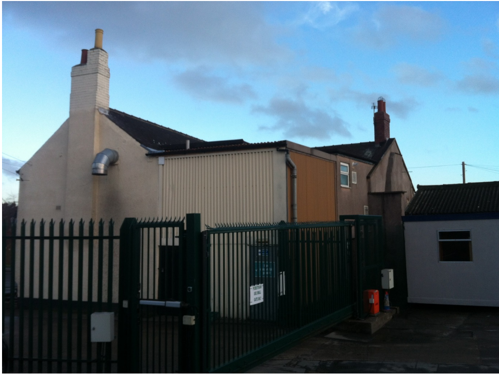
03. Side and part rear elevation viewed from Fosters Bakery Yard.
