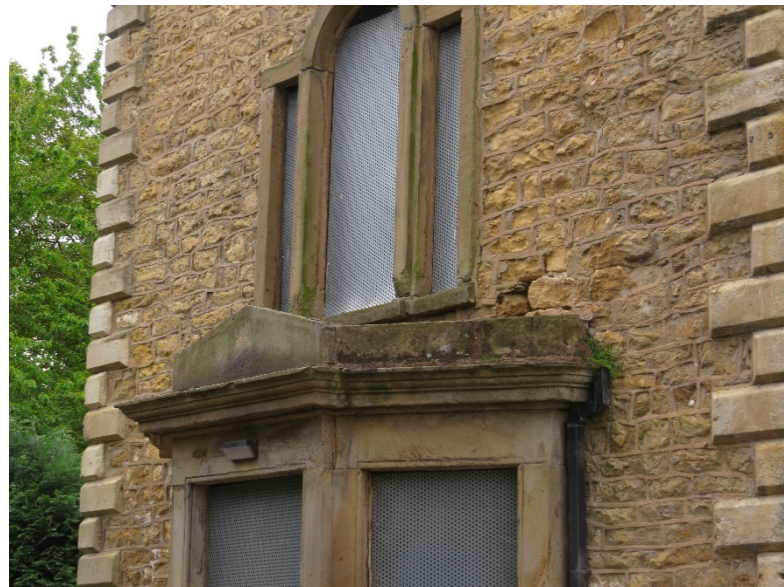
Fig 7 – Bay Window with venetian window over
