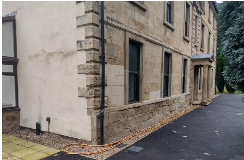
Fig 11: South Façade, historic stonework retained (2 nd storey windows added during conversion to nursing home in the late 20 th Century)
