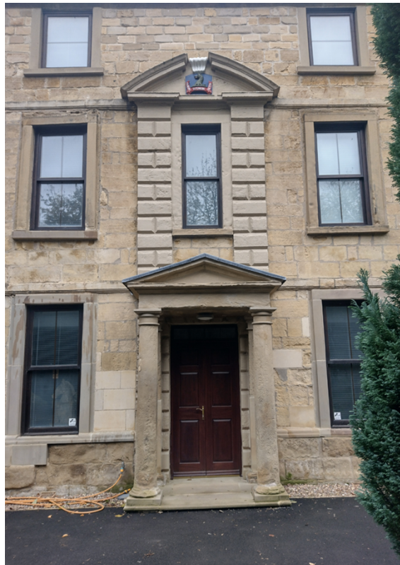
Fig 10: South Entrance and Portico
