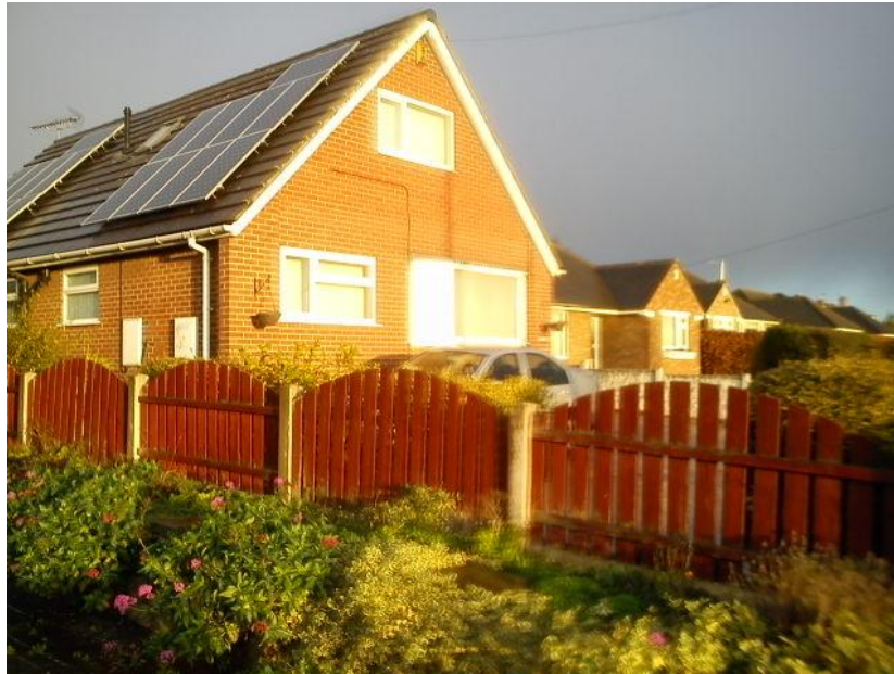
Existing bungalow to the north of the site
