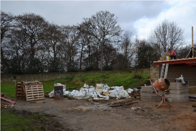
1.0 - P4. View Plot 4 from SE corner
