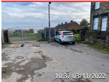
BACK LANE FOOTWAY 8
