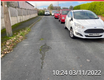
WELL LANE A2
