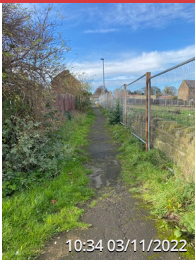
BACK LANE FOOTWAY 4
