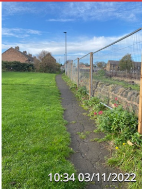
BACK LANE FOOTWAY 3
