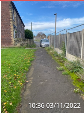
BACK LANE FOOTWAY 6
