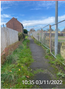
BACK LANE FOOTWAY 5
