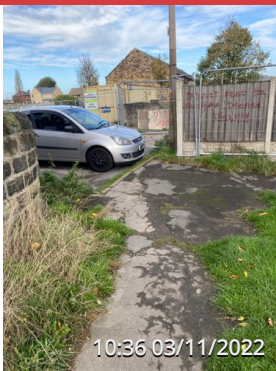
BACK LANE FOOTWAY 7
