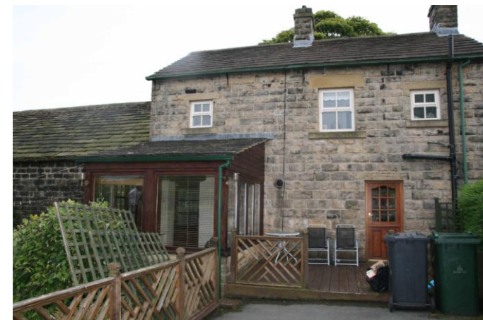
Fig.6 Existing North /Rear Elevation showing the incongruous existing conservatory and rear boundary treatment.
