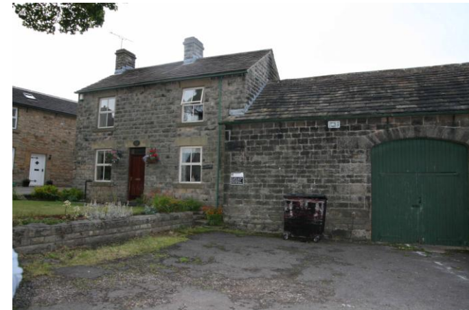
Fig.5 Existing South /Front Elevation showing Stanley House to the West and the storage barn to the East.
