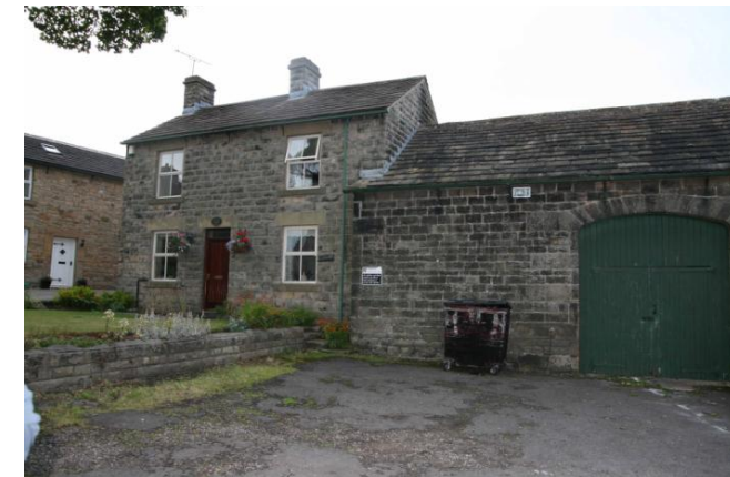
Fig.2 Photo showing Front (South) Elevation. Stanley House to the West and the barn to the East. The area in front of the barn is in separate ownership.
