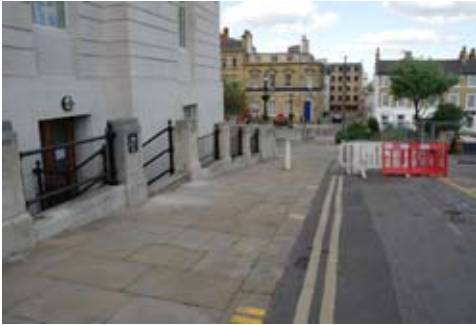
Yorkstone paving and kerbs, southern frontage
