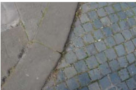
Green/grey granite setts with Yorkstone kerbs
