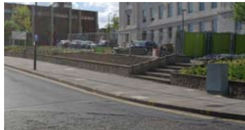
Wide pavements along adjoining highway on Shambles Street
