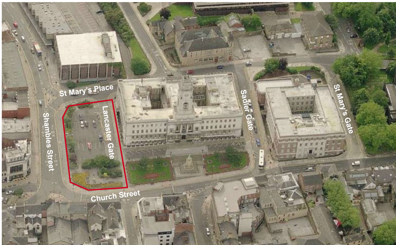
Aerial view of Town Hall from the east showing site boundary
