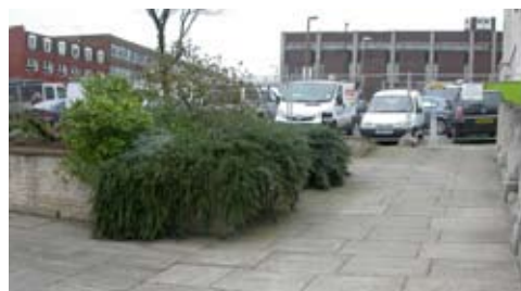
Poorly defined boundary to parking area. Vehicles dominate views along southern frontage
