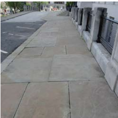
Large Yorkstone paving slabs, eastern Town Hall frontage
