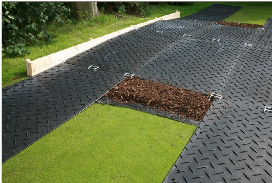
Figure 3. An example of suitable temporary ground protection spanning over a root protection area.
