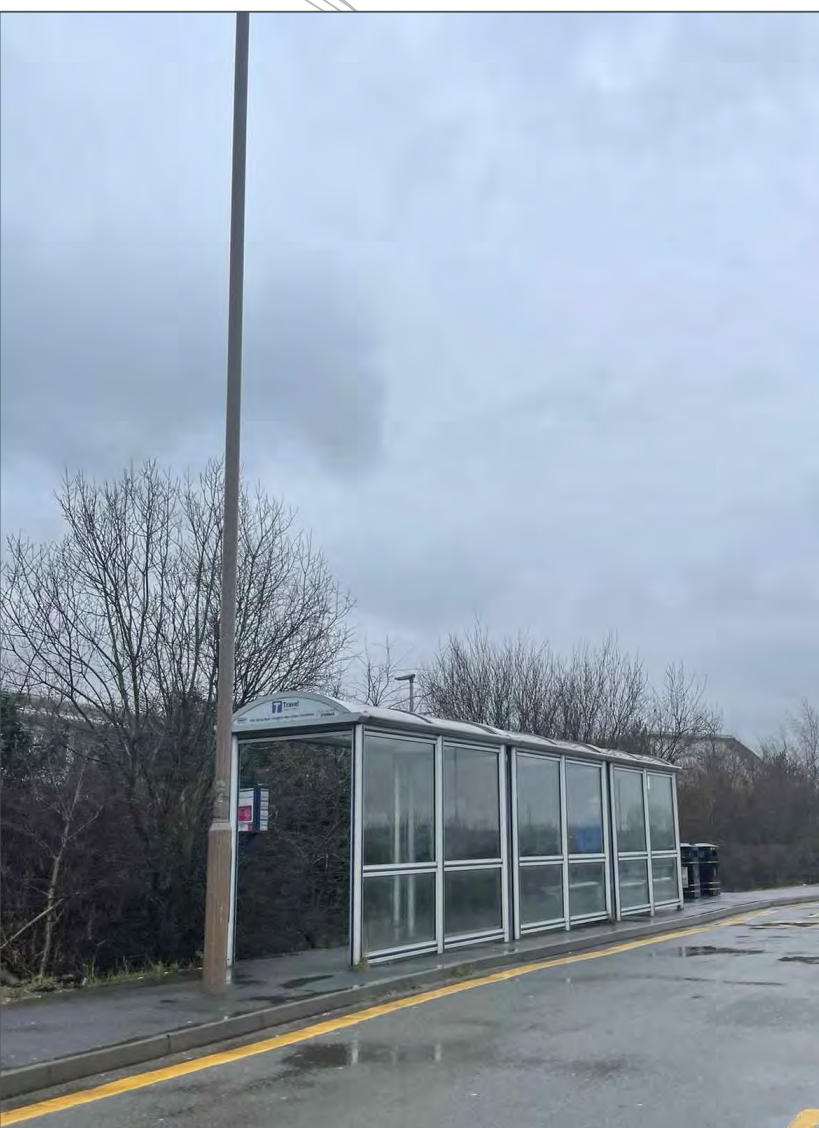
Bus stop with shelter and layby located along Park Spring Road – Photo taken facing South
