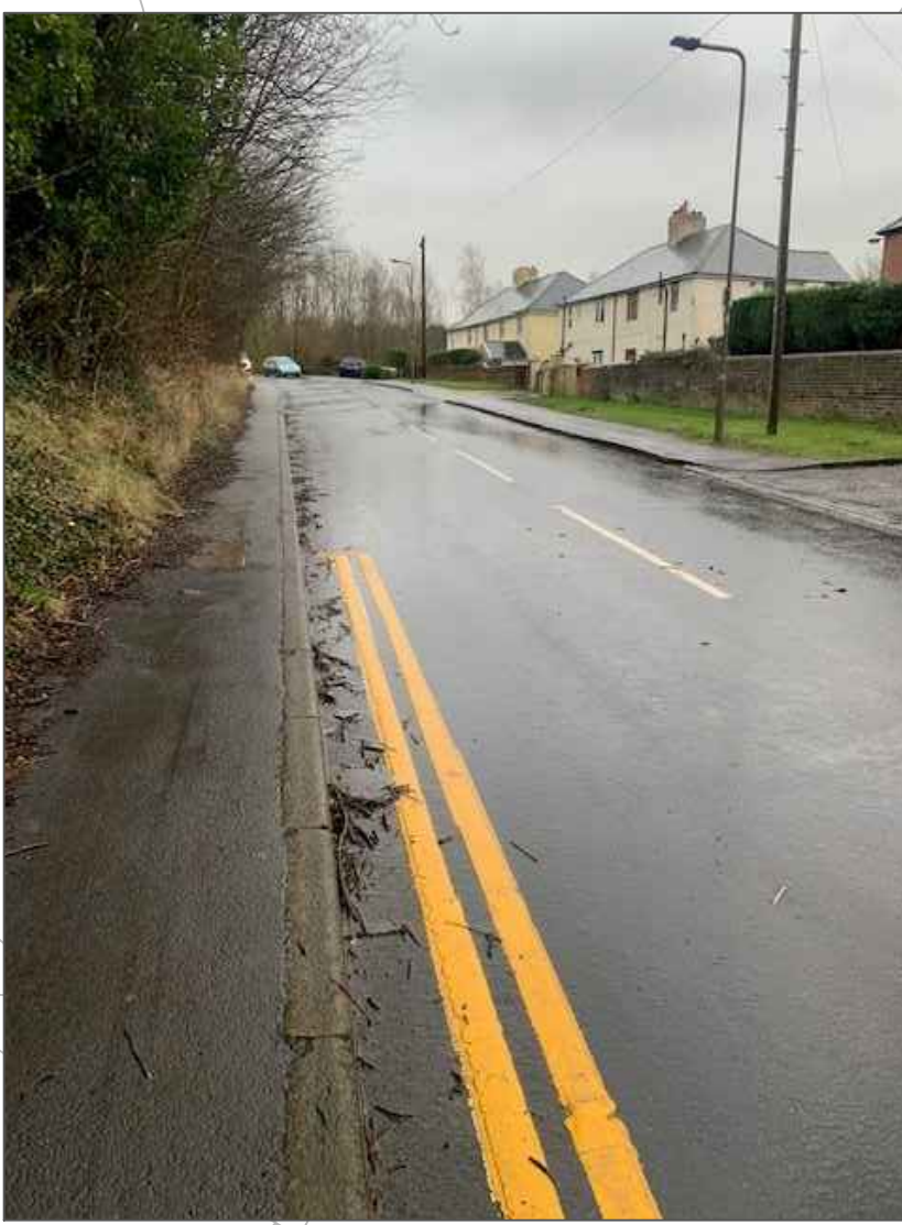
Footways provided on either side of Middlecliffe Lane for the entirety to a minimum width of circa 1.3m – Photo taken facing South East
