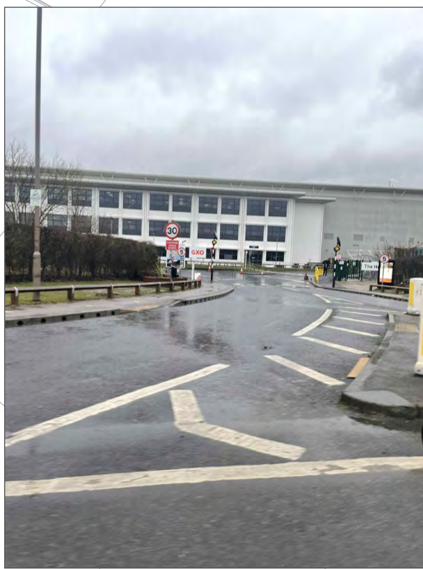
Dropped crossings and pedestrian refuse areas on all arms of the roundabout – Photo taken facing East
