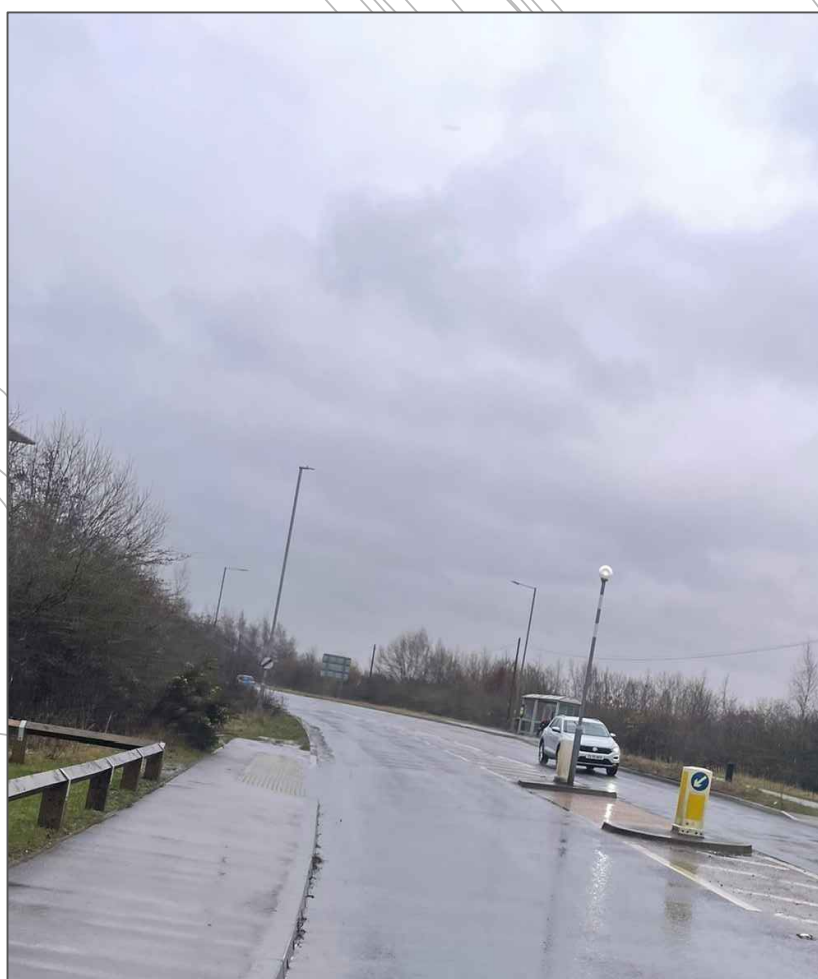
Crossing point with dropped kerbs, tactile paving and central island where southbound carriageway footpath ends. Allows crossing to NB bus stop – Photo taken from South
