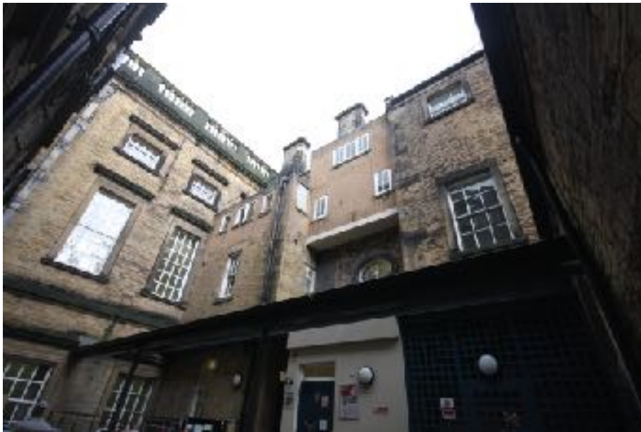
Courtyard showing location of new outlet and the rainwater pipe which is to be replaced (alongside an existing soil and vent pipe).
