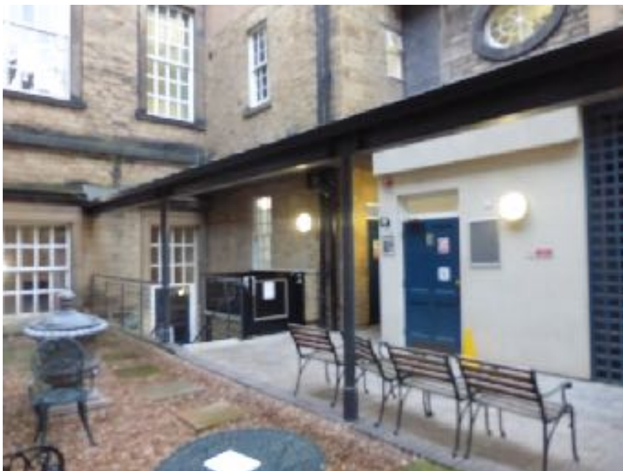
Courtyard at low level showing existing soil and rainwater pipes.
