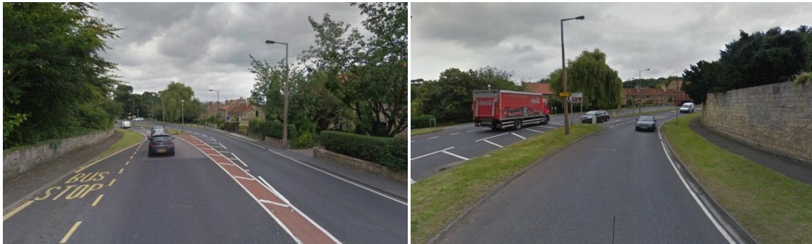
PP5: Second exit of a roundabout on the A635.
