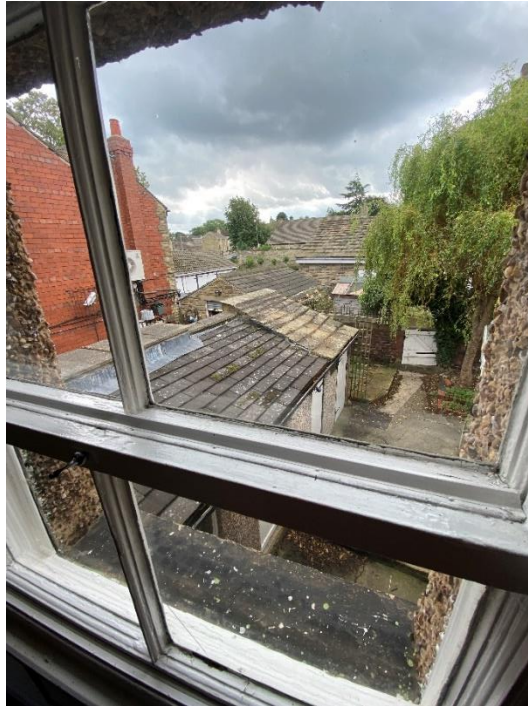
Figure 21 Showing the view from the first floor out over the rear court yard of 1 Maltkiln Row.
