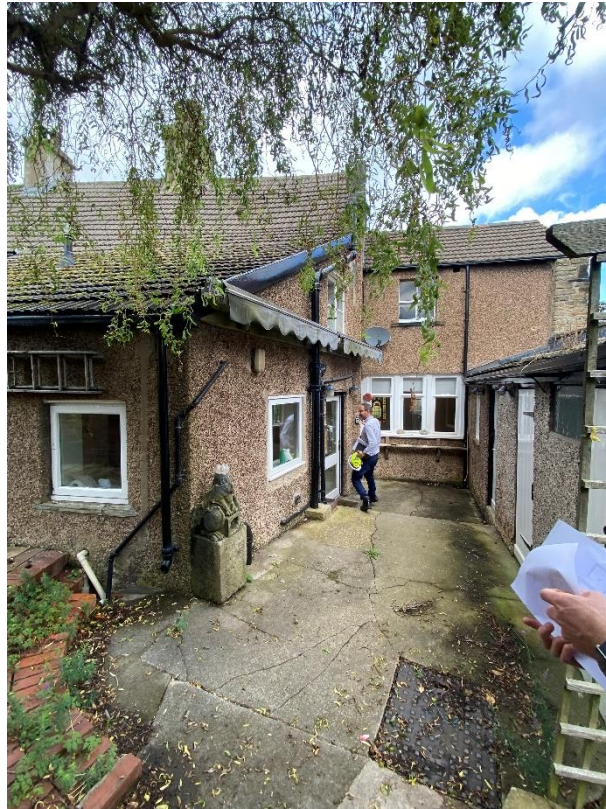
Figure 19 Showing the rear of 1 Maltkiln Row.
