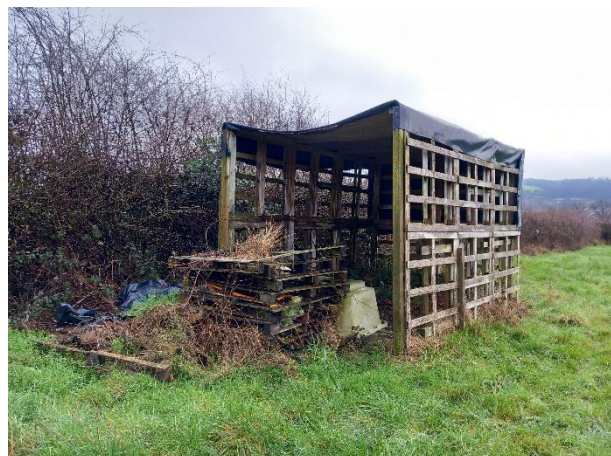
Photograph 14: Structure in north-western field, made of pallets (Figure 1, TN).
