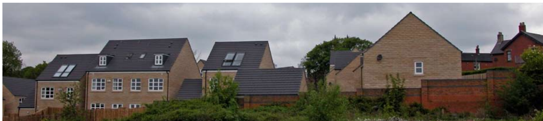
artificial stone and slate sited next to red brick dwelling
