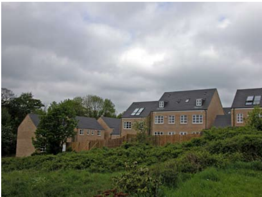
Housing on the site of the former Dodworth C of E School has been constructed in artificial stone with slate roofs.
