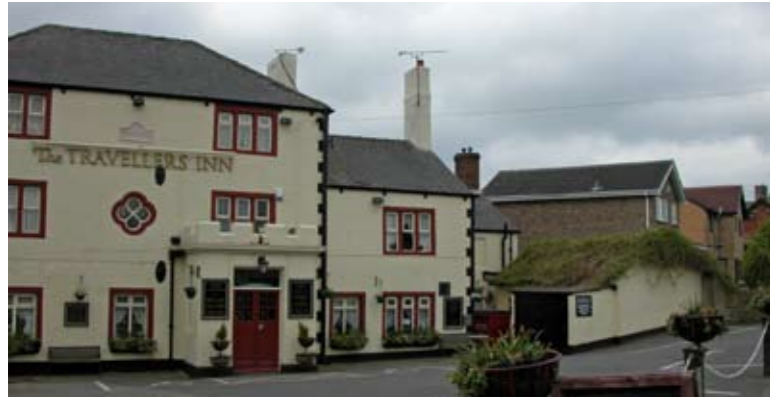
render / slate roof sited next to brick property
