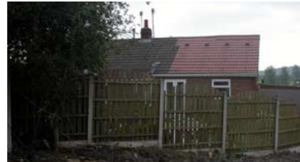
grey tile roof - extension completed in red tile
