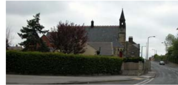
church constructed in traditional stone and slate roof
