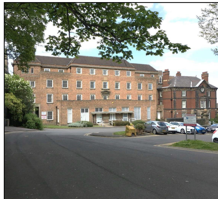
Above: Existing office building and building to be retained (on left)
