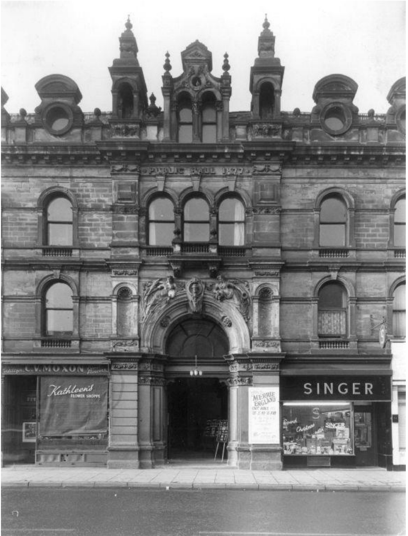
Fig. 24: Archive Image of Entrance 1963
