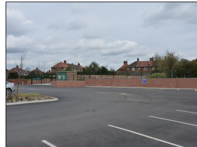
VIEW FROM HIGH STREET ONTO SITE
