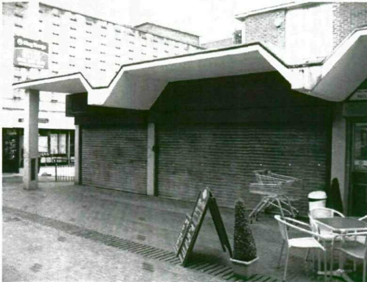
Frontage to Market Street
