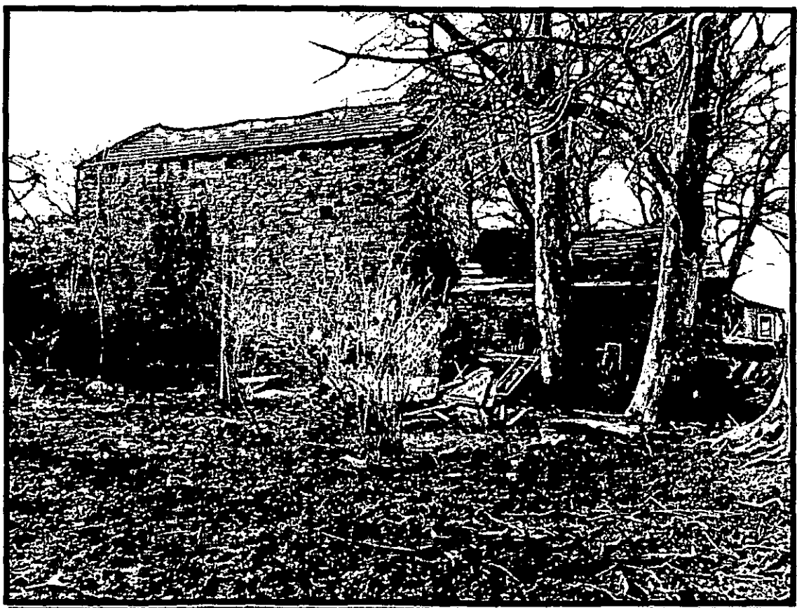
Photograph 50 – View of East Elevation showing trees
