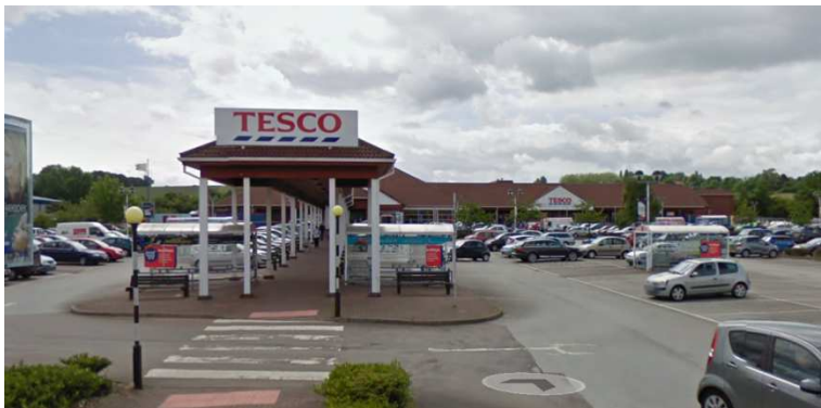
View of Tesco Store and Walkway
