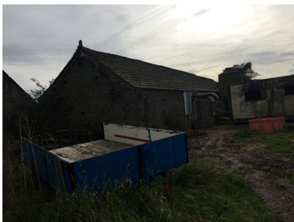
Plate 3 West aspect of Building 1
