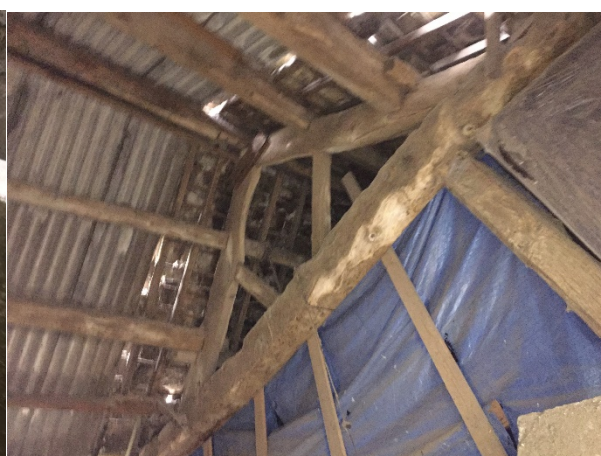
Plate 10 Detail of interior roof of Building 1
