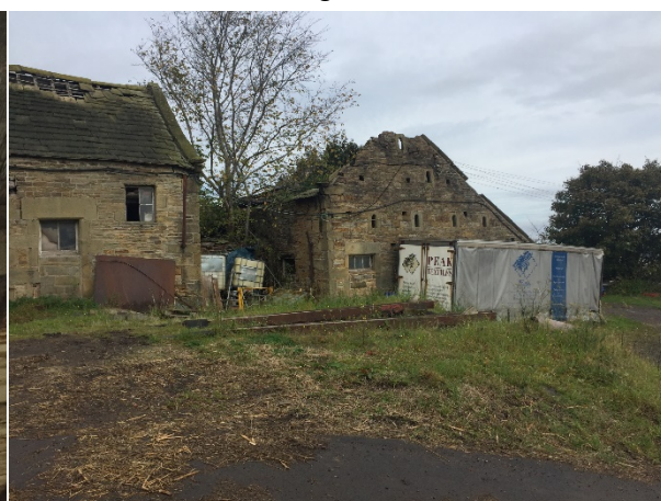
Plate 18 South aspect of Building 3
