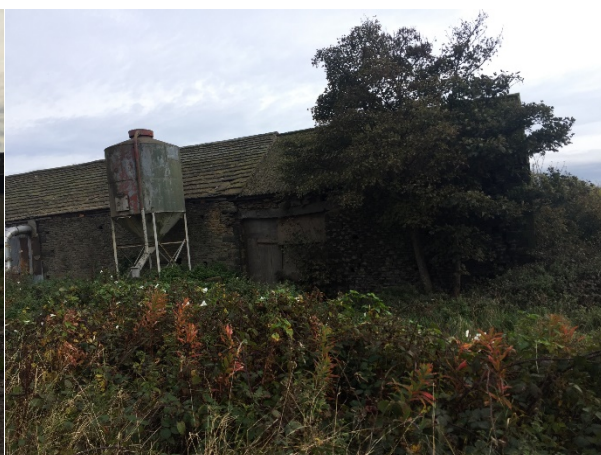
Plate 4 West aspect of Building 1
