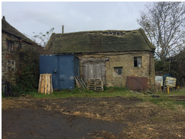
Plate 13 South aspect of Building 2
