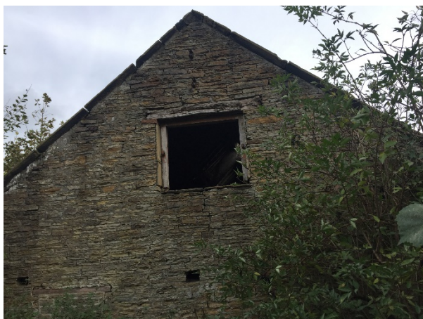
Plate 15 West aspect of Building 2
