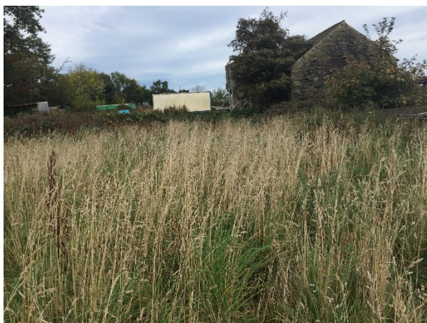
Plate 5 South gable of Building 1
