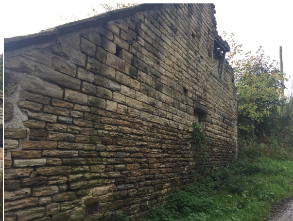
Plate 20 North aspect of building 3
