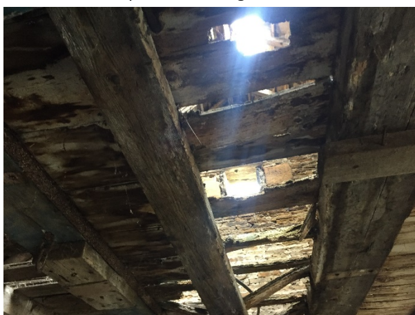
Plate 17 Detail of ceiling in Building 2
