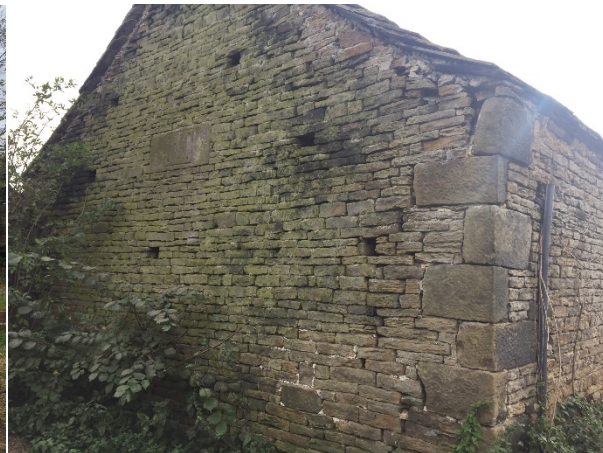
Plate 14 Northwest aspect of Building 2
