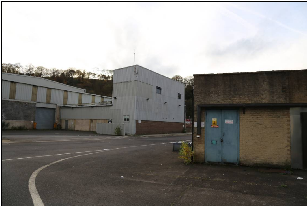
Plate 4: A view from the eastern bank of the River, looking west. Most of the large, mid 20th-century industrial sheds survive, but are of little architectural or historic interest.
