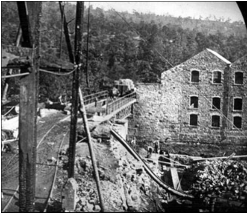
Plate 1: A photograph taken from the surviving warehouse building (HA1), showing the later buildings on the eastern side of the Don, of which the lower walling survives (HA4). It is likely that the photograph was taken following the 1899 fire, as building debris is seen in the foreground (in the centre of the yard) (Picture Sheffield, s09931).
