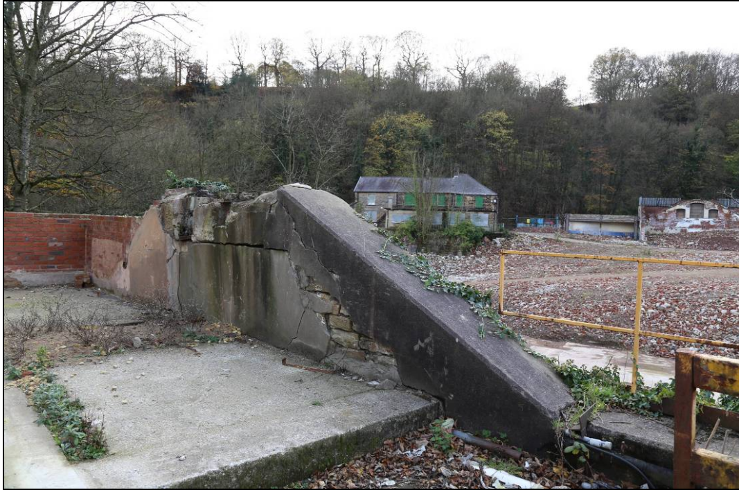
Plate 5: A general view of the site taken from the platform on the east bank of the River Don (showing the rear of HA4 ), looking west. It shows the extent of demolition and building HA3 in the background.
