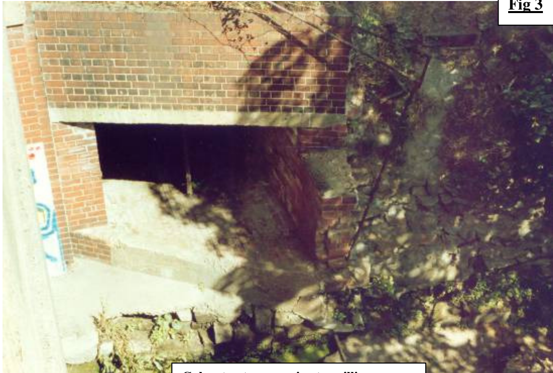
Culvert entrance prior to grilling.
