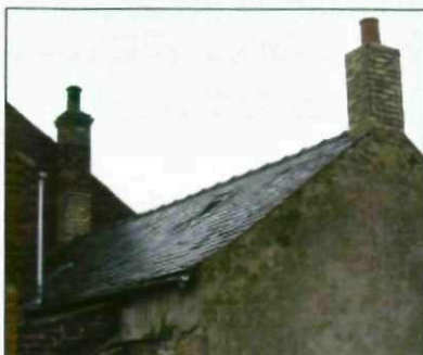
The East roof slope
