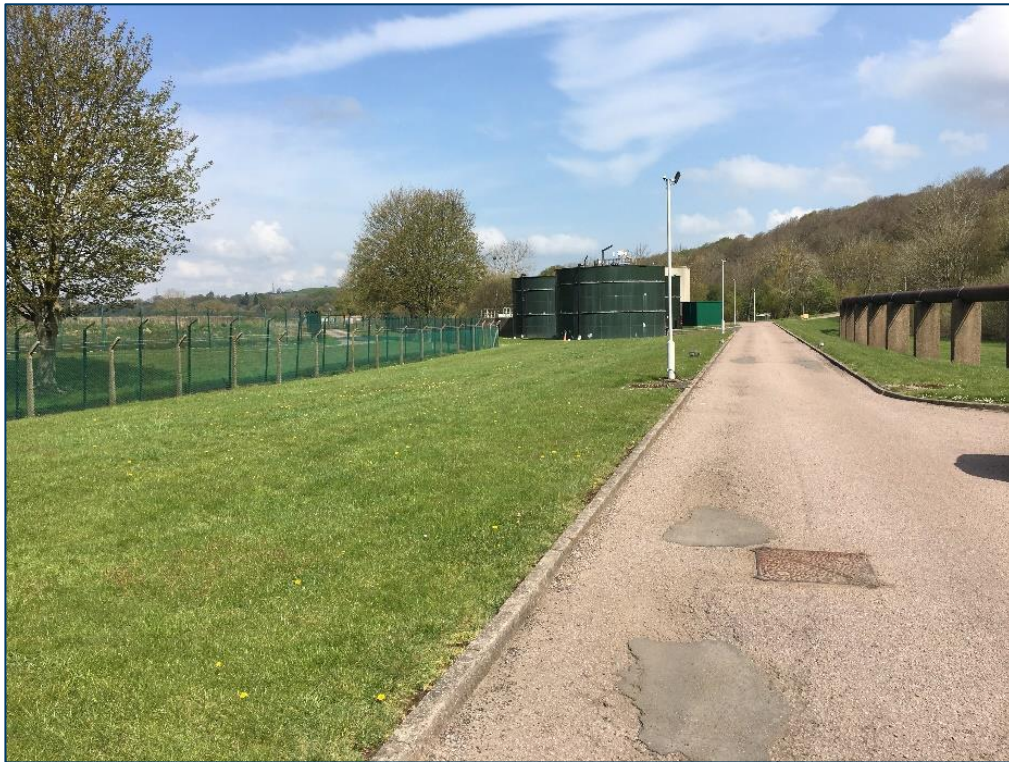
Figure 2 Site ground level facing northwest across the site.
