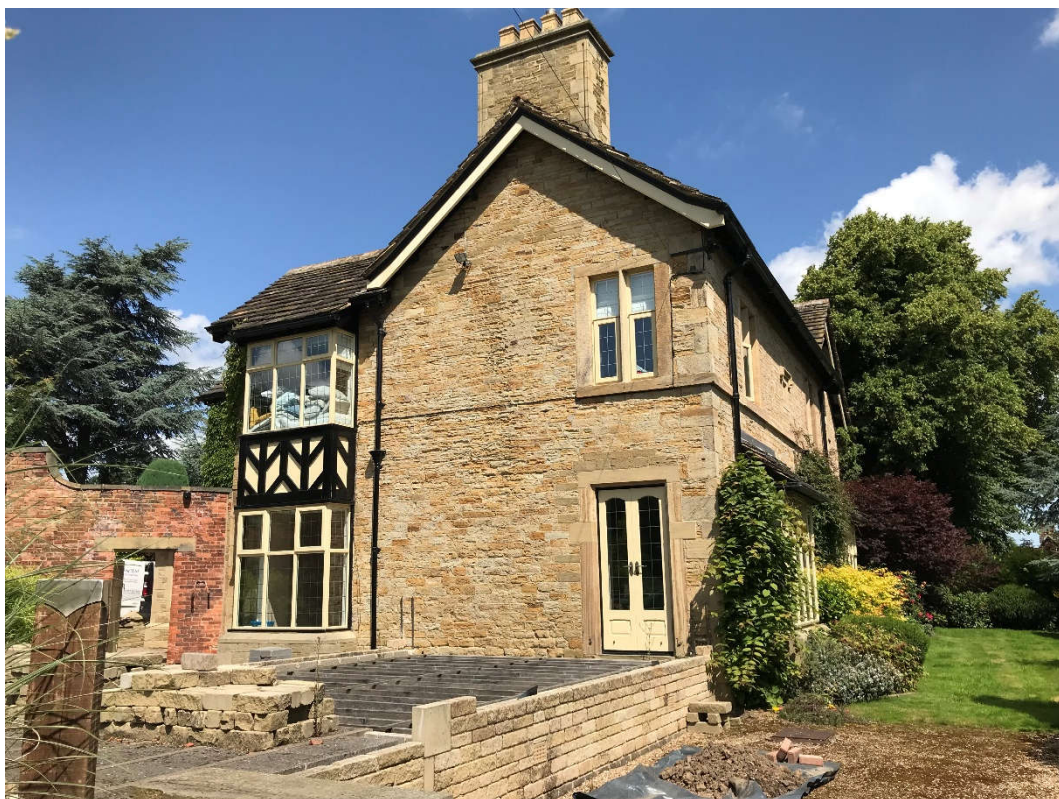
Fig 10. South gable of Dale House – shows commencement of development of former approved single storey side orangery extension.
