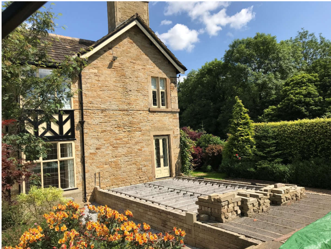
Fig 09. South gable wall of Dale House – location for two storey extension.
