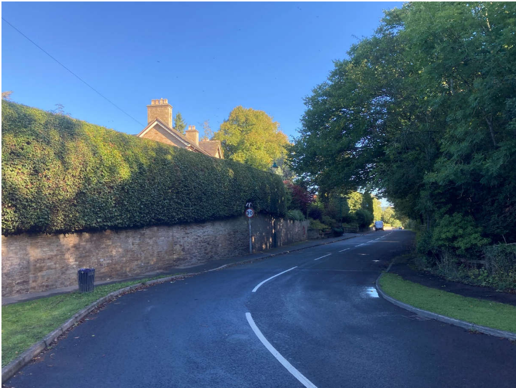
Fig 02. View of Dale House frontage from the junction of Lane Head Road.
