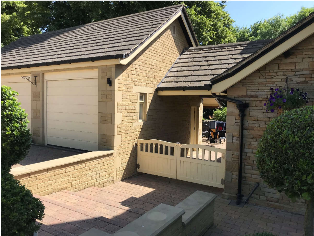
Fig 07. View of south garage gable and open link roof to house.
