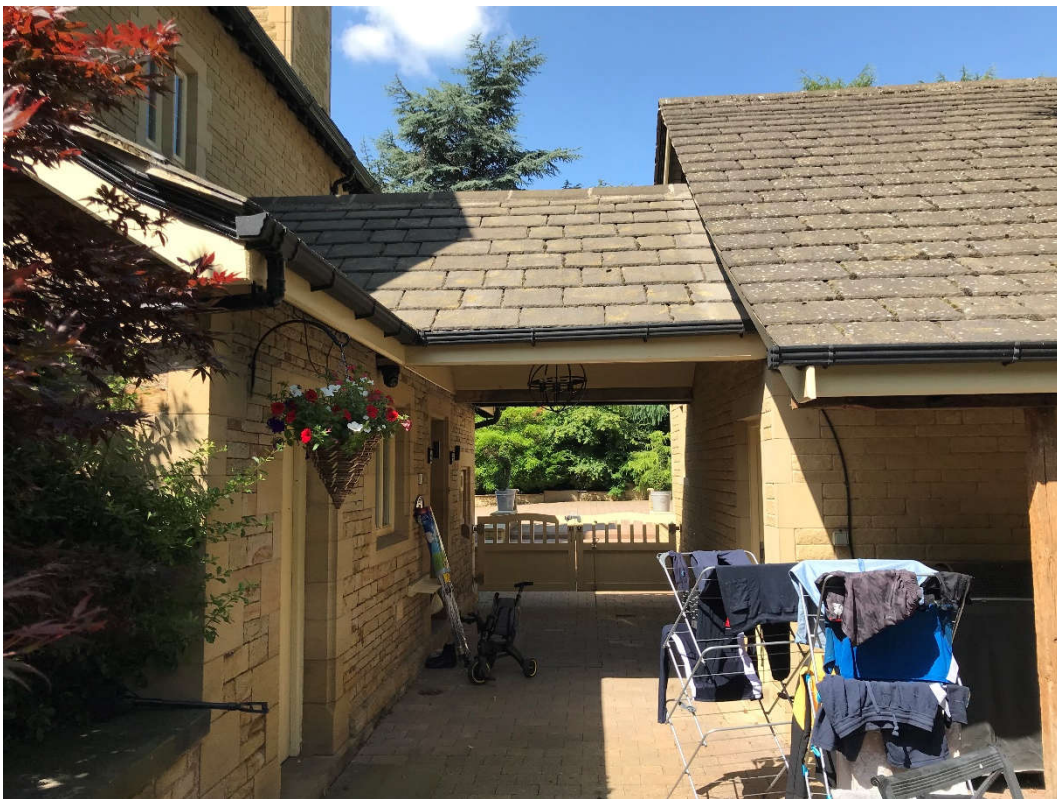
Fig 08. View of existing link roof between house and garage looking west.
