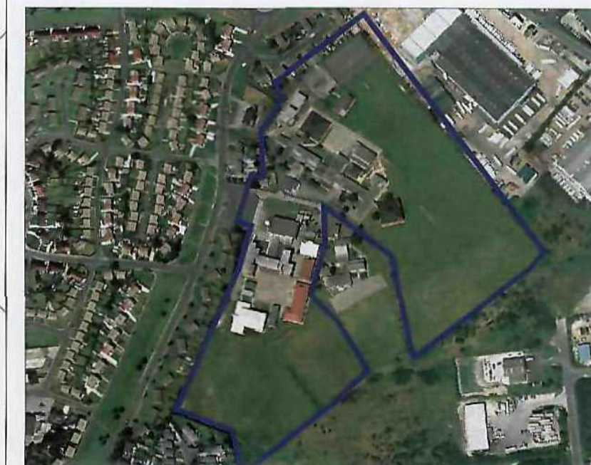
AERIAL VIEW OF EXISTING SITE
