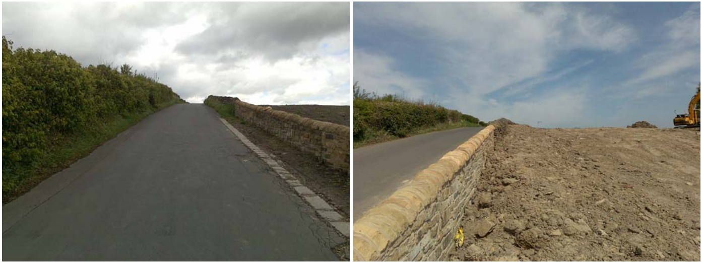
Photos 2 & 3 – Stone Wall adjoining Bromley Carr Road
