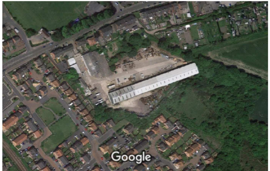
Existing Premises at 321 Haugh Lane, Wombwell
